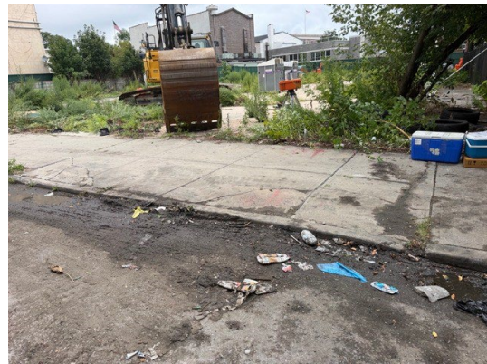
Excavator seen from Beach 19 th Street
