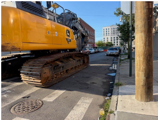
Excavator arriving at site
