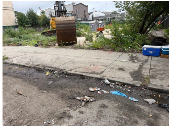
Excavator seen from Beach 19 th Street
