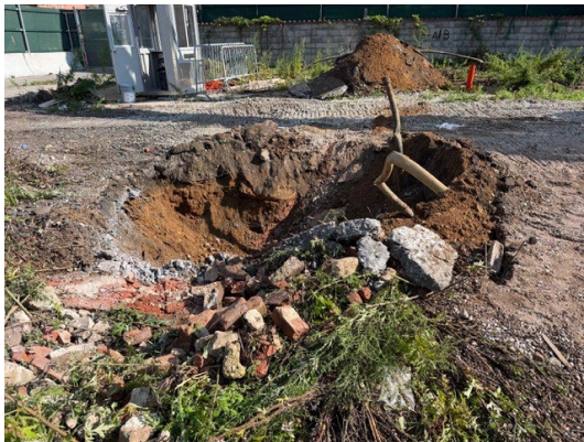
Test pit (fuel line for suspected storage tank encountered), Grid A2
