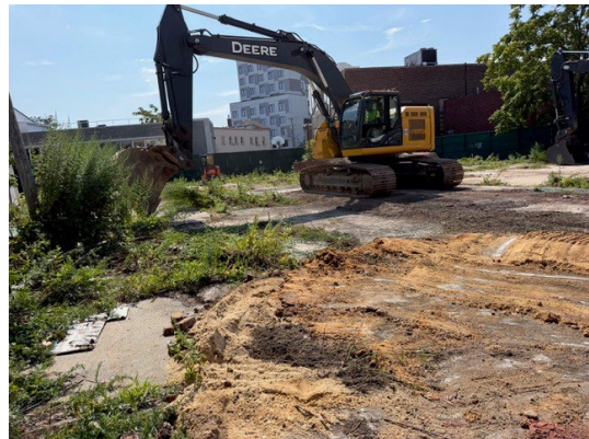
Waste characterization test pit, Grid D1
