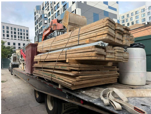
Material delivery to the site
