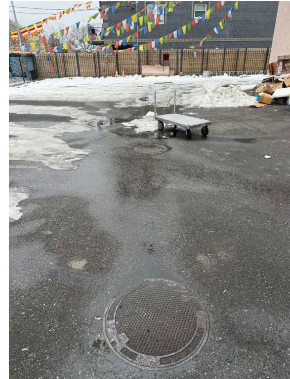
View of manholes of retention tank system beneath the open parking area
