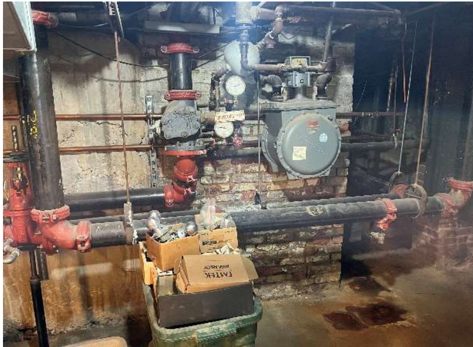
Photo 11: Water meter and sprinkler system within the eastern portion of the basement of the subject property.
