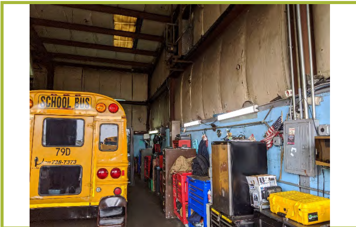
Photo #9: Interior finishes in Maintenance Garage.
