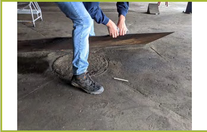
Photo #7: Manhole cover observed in Maintenance Garage.
