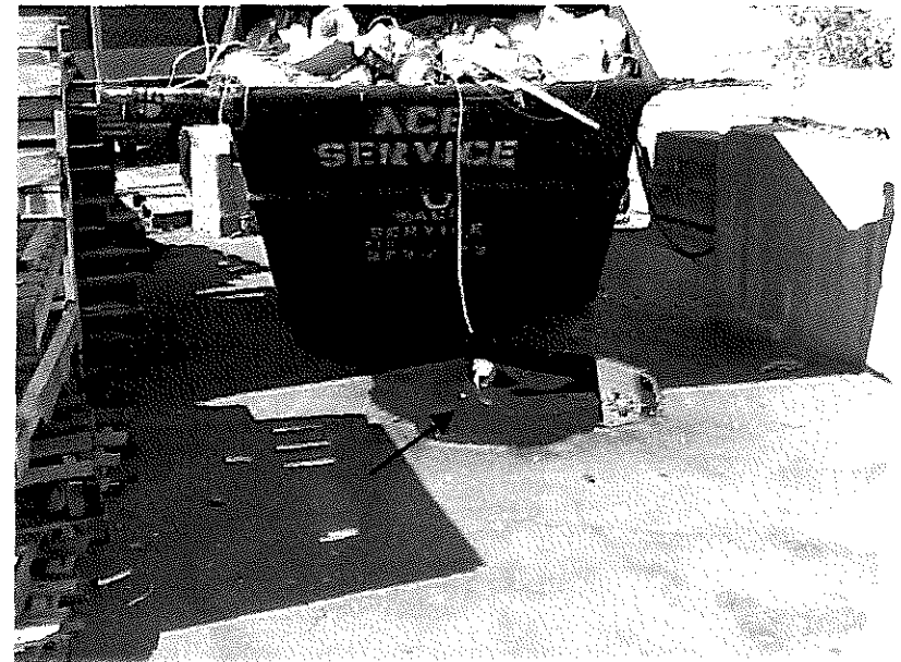
Picture #24: View of the on-site drywell (arrow) and former trench area (in background) in the parking area on-site.
