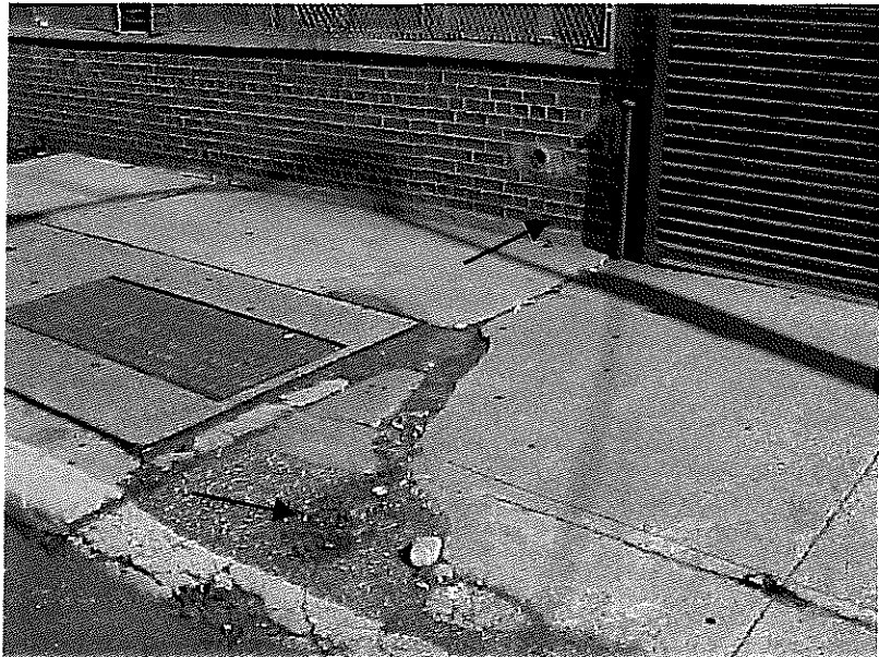
Picture #13: View of the fill caps and vent pipe associated with a former fuel oil tank closed in-place on the subject property.
