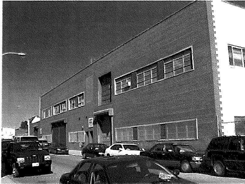
Picture #1: View of the building located on the subject property.
