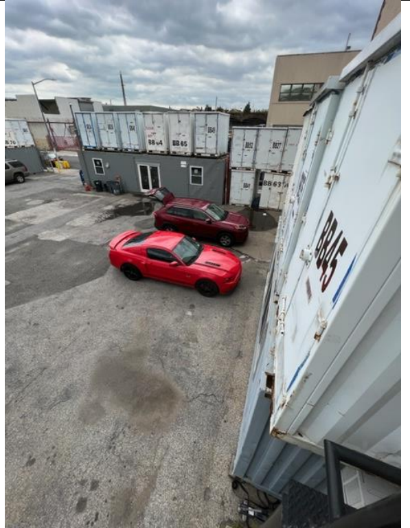
View of Subject Property Parking Lot from the Roof
