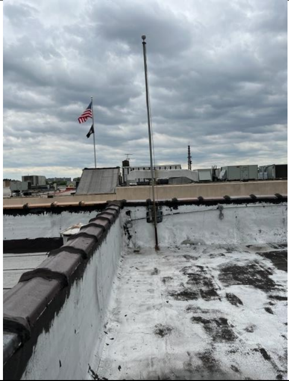
Subject Property Roof
