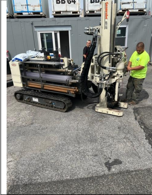
Soil Probe Installation at Subject Property
