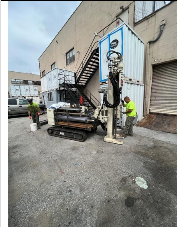
Soil Probe Installation at Subject Property
