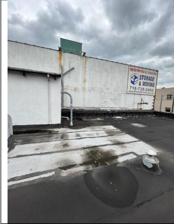
Subject Property Roof
