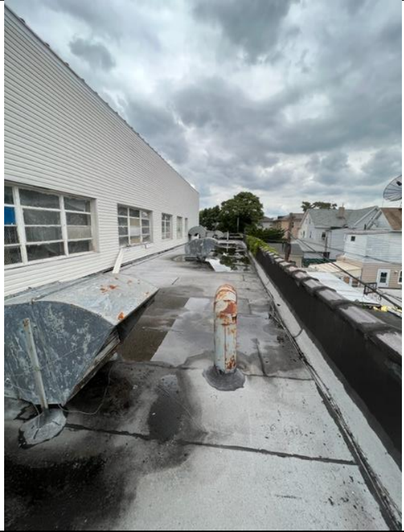
Subject Property Roof
