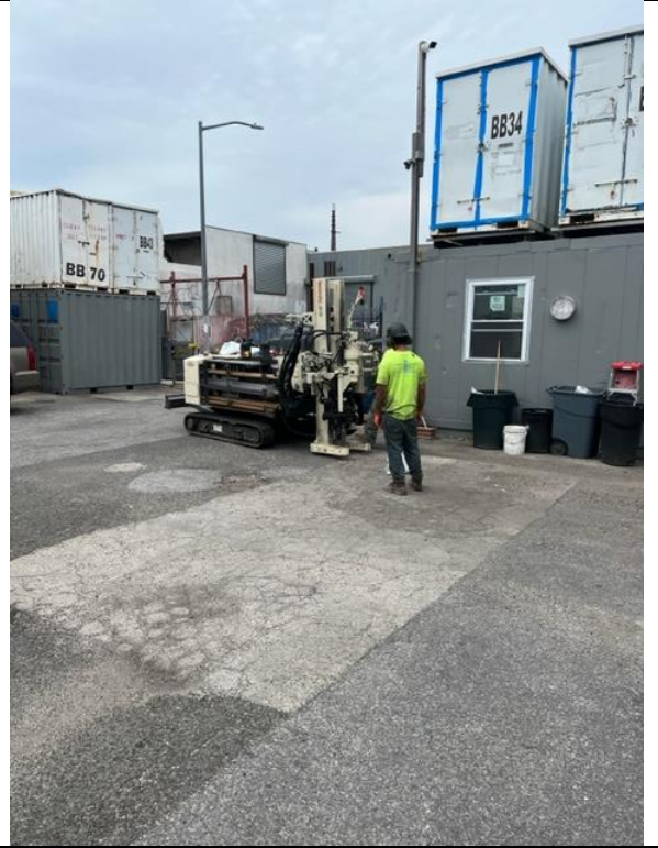
Soil Probe Installation at Subject Property
