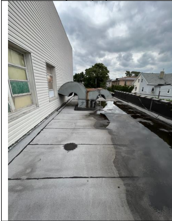
Subject Property Roof
