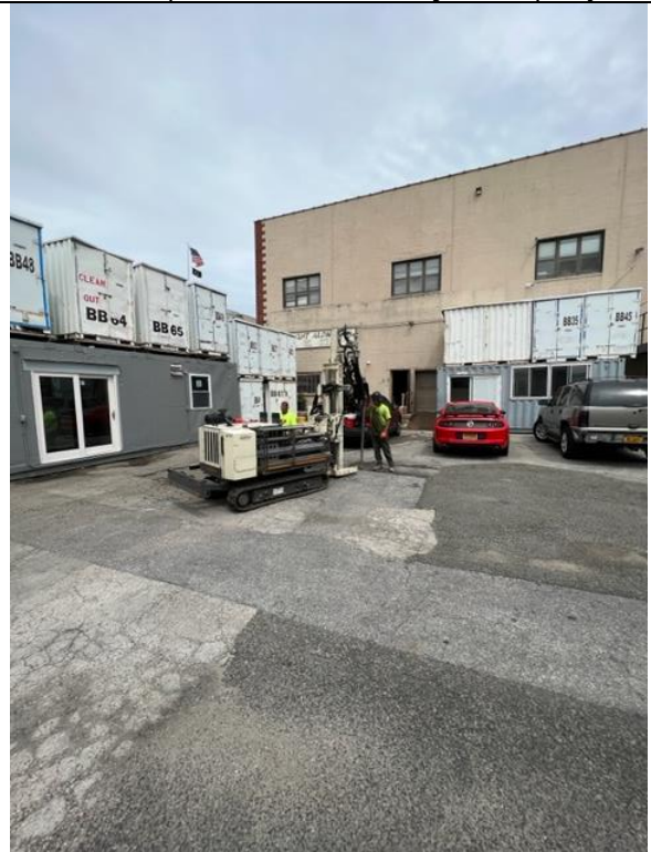
Soil Probe Installation at Subject Property
