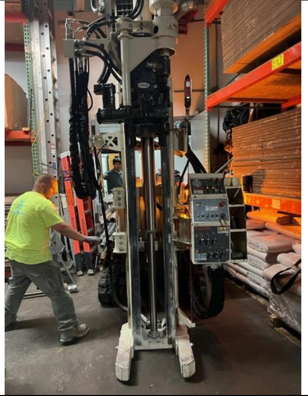
Soil Probe Installation at Subject Property
