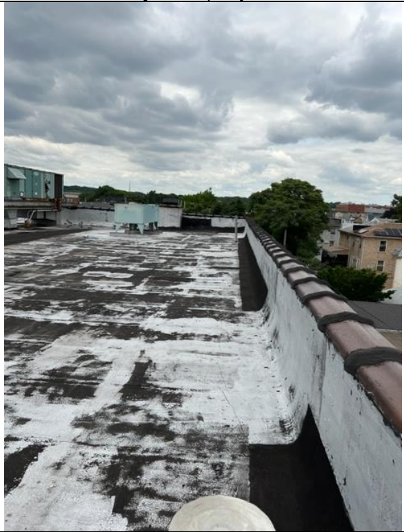
Subject Property Roof
