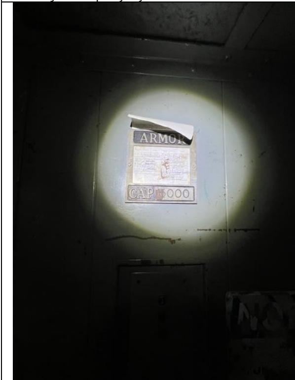
Subject Property Hydraulic Elevator Certificate
