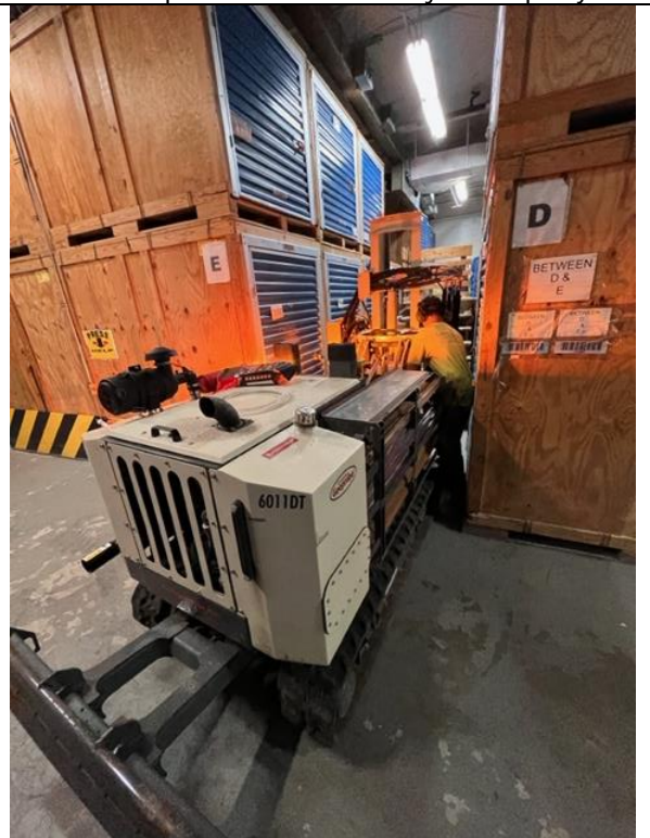
Soil Probe Installation at Subject Property
