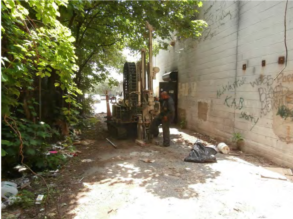
Photo 4 – Drilling soil boring B-2 in the northern portion of parking lot.
