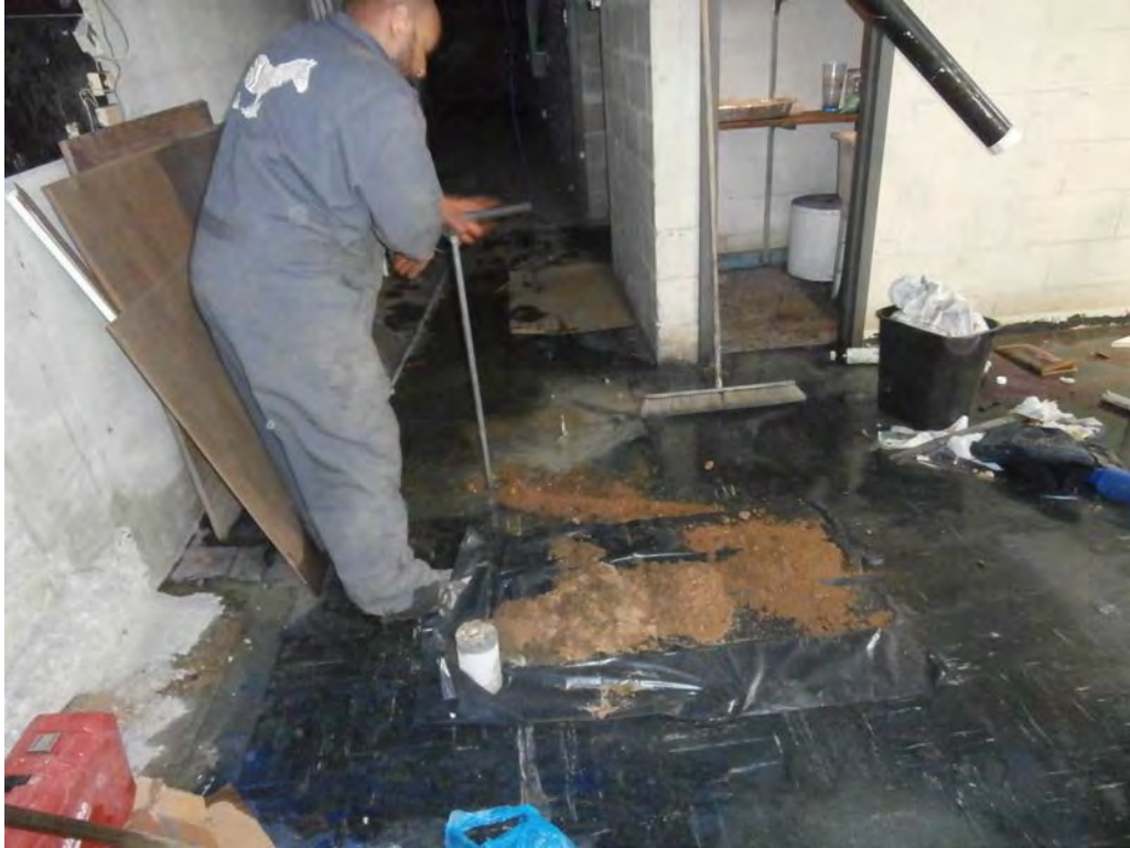
Photo 3 – Zebra hand drilling B-1 in basement.
