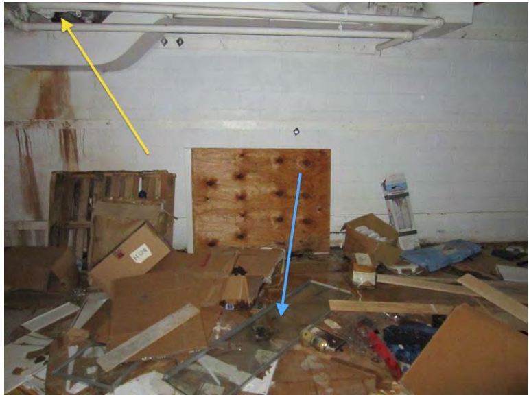
The yellow arrow points towards the possible source of a significant water leak, and the blue arrow points towards standing water on the floor and water-soaked materials. A strong musty/moldy odor was noted in this basement.
