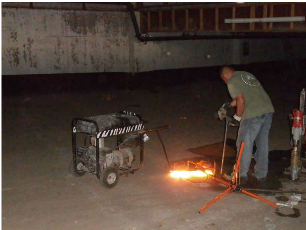
Photo 11 – Zebra hand drilling B-8 in southern section of garage near location of former UST.
