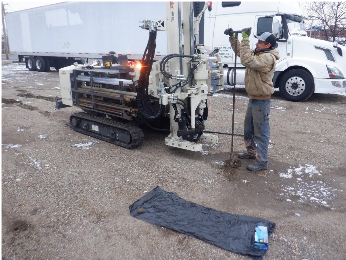
Photograph No. 1 & 2: View of drill technician hand-clearing sampling locations prior to utilization of a remote access rig to complete soil borings on the subject property located at Beach 62nd St, Queens, NY.
