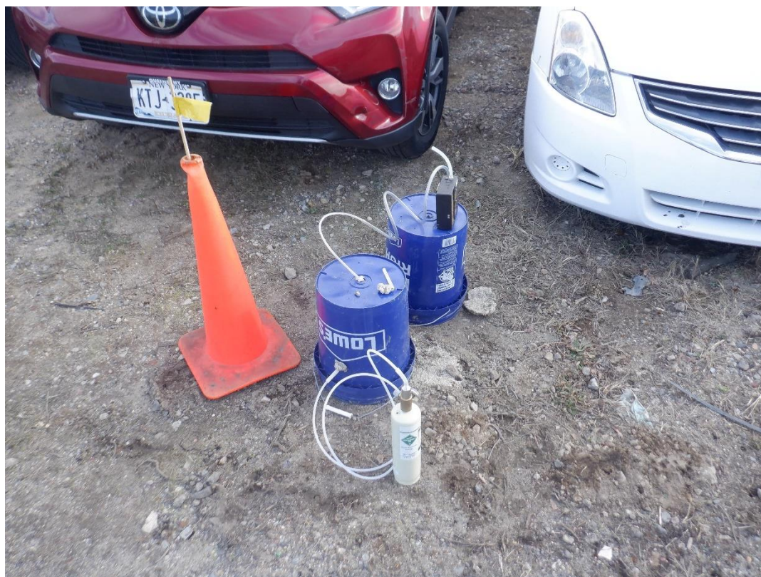
Photograph No. 6: View of one (1) sub slab soil vapor sample collection from the subject property during the investigation.
