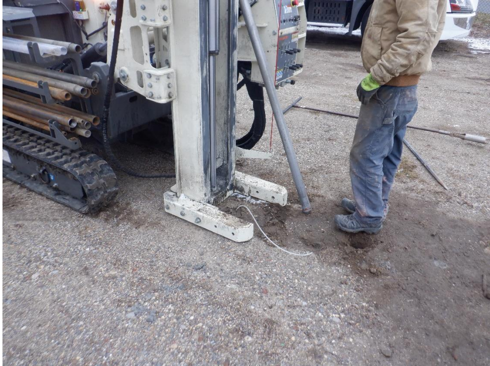
Photograph No. 3: View of soil boring that was converted into a temporary soil vapor monitoring location.
