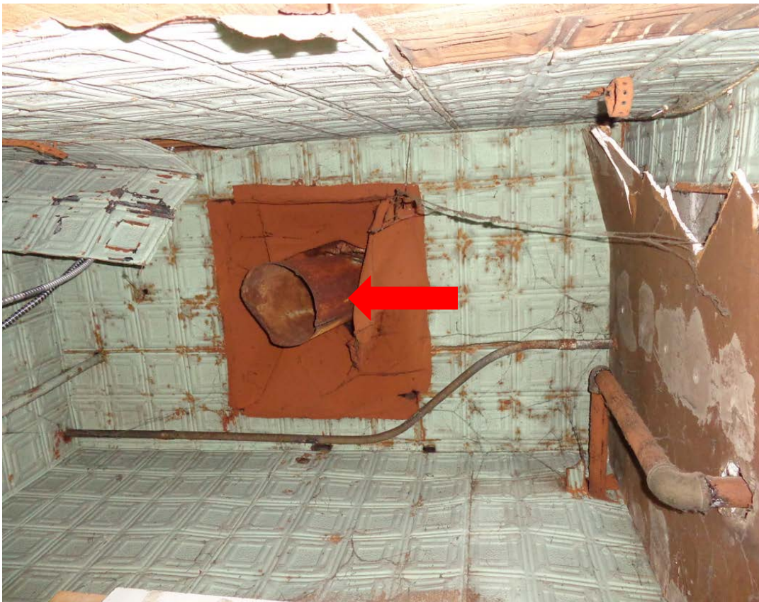
Figure 10: View of the suspected ceiling vent within the current Laundromat for either a boiler or dry cleaning equipment that was determined to have operated on-site.
