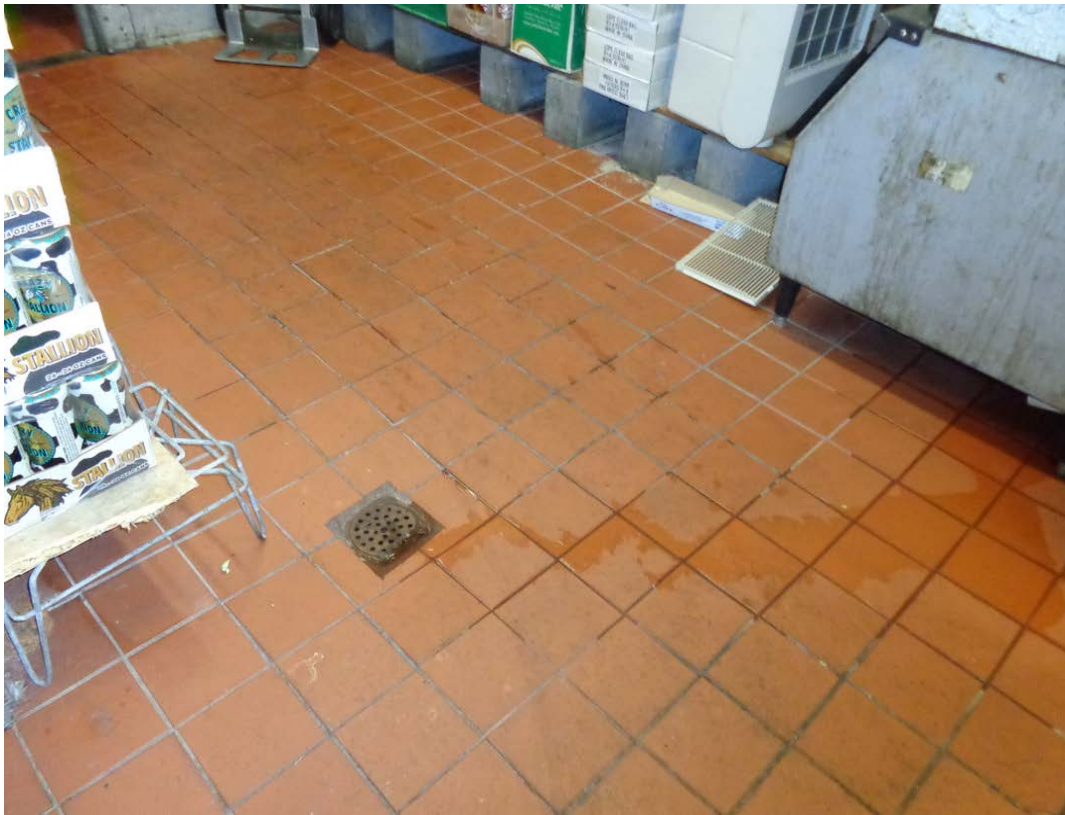
Figure 5: The grocery/supermarket on-site includes interior floor drains. No hazardous materials were observed entering into these interior floor drains.
