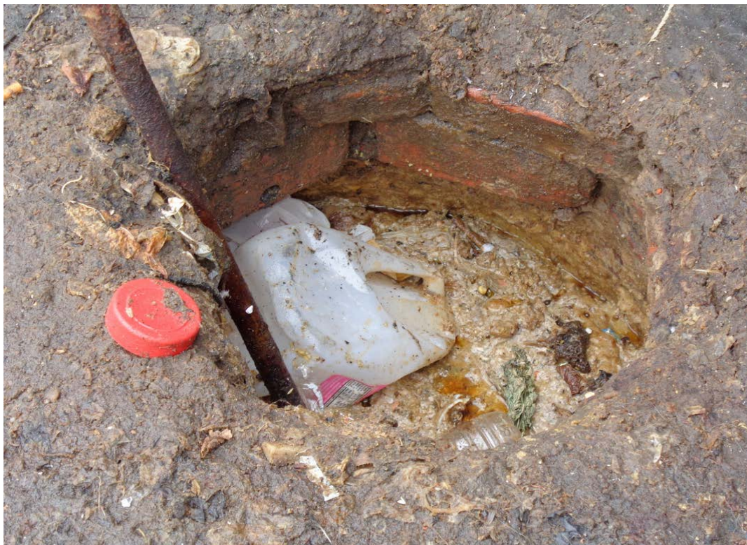
Figure 14: Close up view of the open drain within the parking lot on-site.
