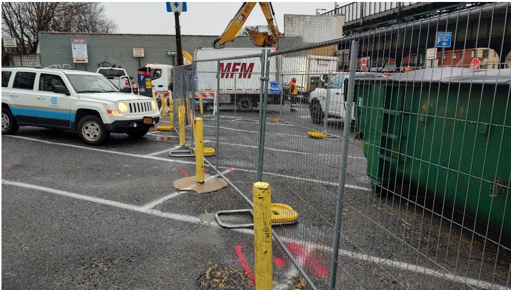
Photos 4 & 5 – Location of the center of the parking lot with the detected electrical lines leading to the parking meters and site lighting, marked in red.
