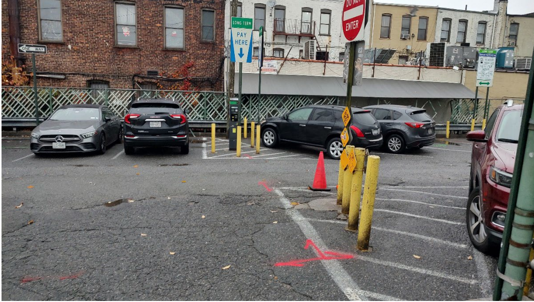
Photos 4 & 5 – Location of the center of the parking lot with the detected electrical lines leading to the parking meters and site lighting, marked in red.
