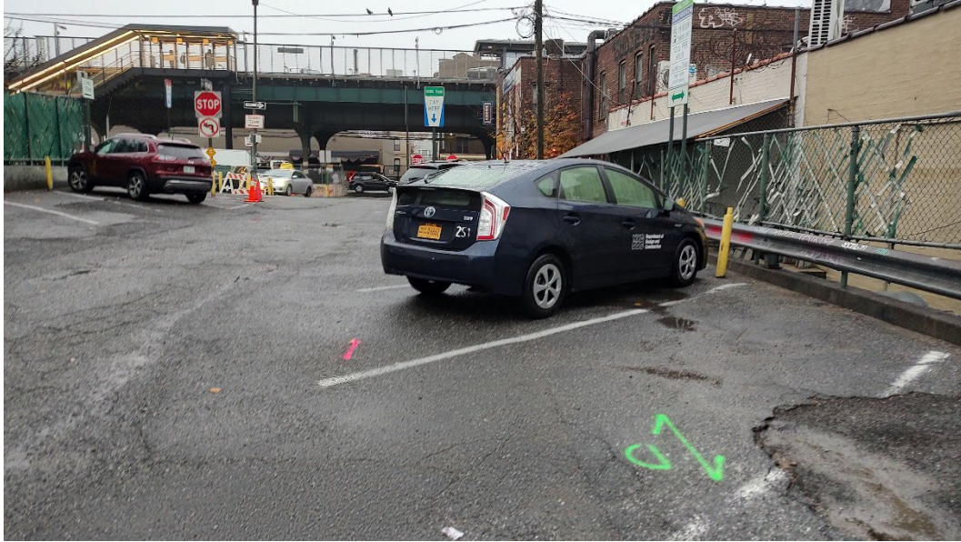
Photos 2 & 3 – Location of the northeastern side of the parking lot containing the storm drain line marked in green and the partial markings of the unknown line marked in pink.
