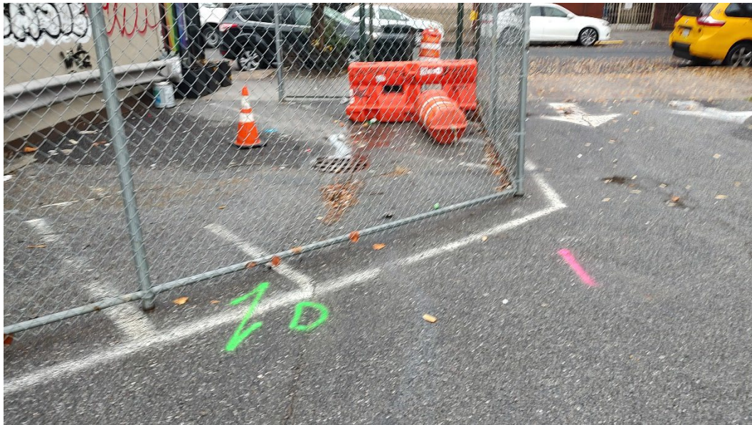
Photos 2 & 3 – Location of the northeastern side of the parking lot containing the storm drain line marked in green and the partial markings of the unknown line marked in pink.
