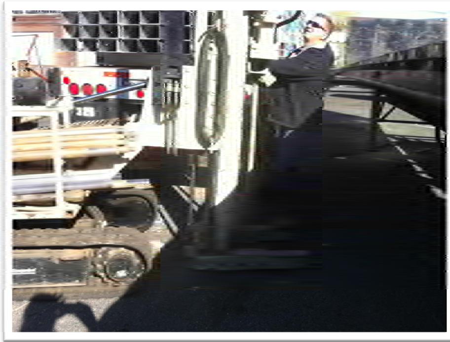
3. Geoprobe Equipment- Soil and Ground Water Borings
