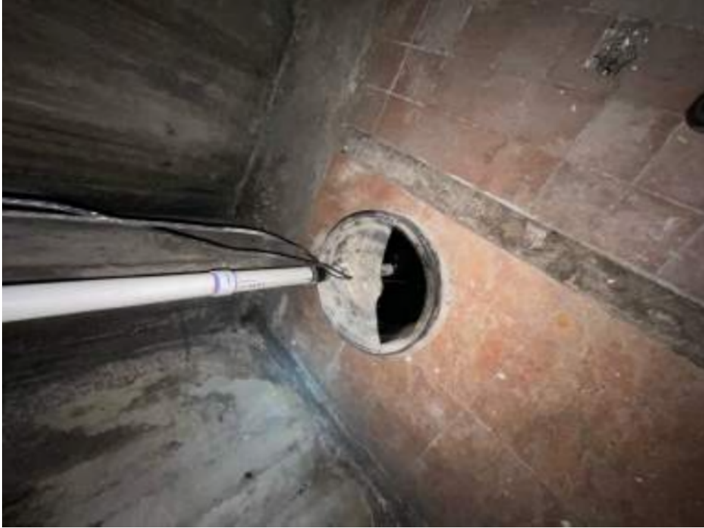
Sump in basement floor
