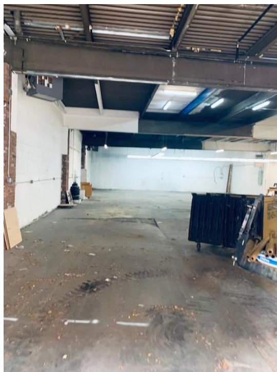
Clearing boreholes inside
