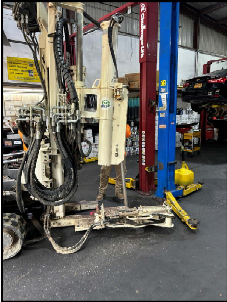
Typical view of the Geoprobe installing a temporary monitoring well.
