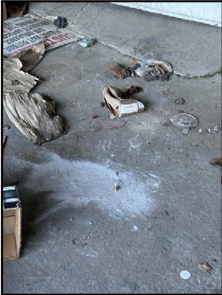
Typical view of a soil vapor point installed using Vapor Pin.
