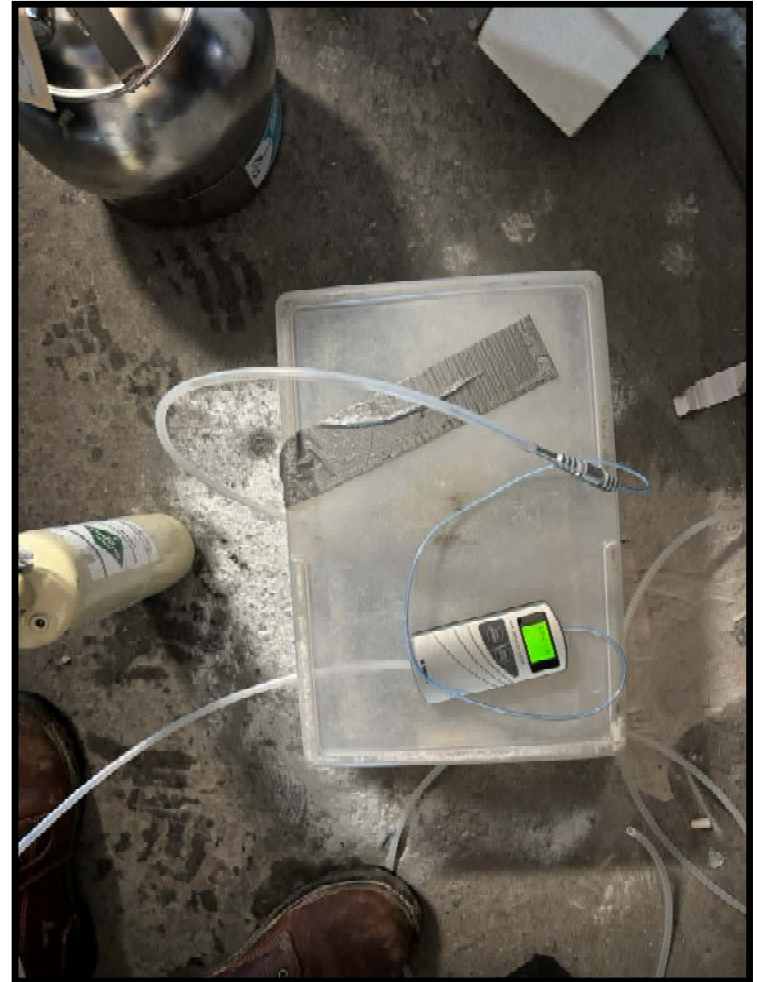
Typical view of the leak test using helium gas being conducted at a soil vapor point.
