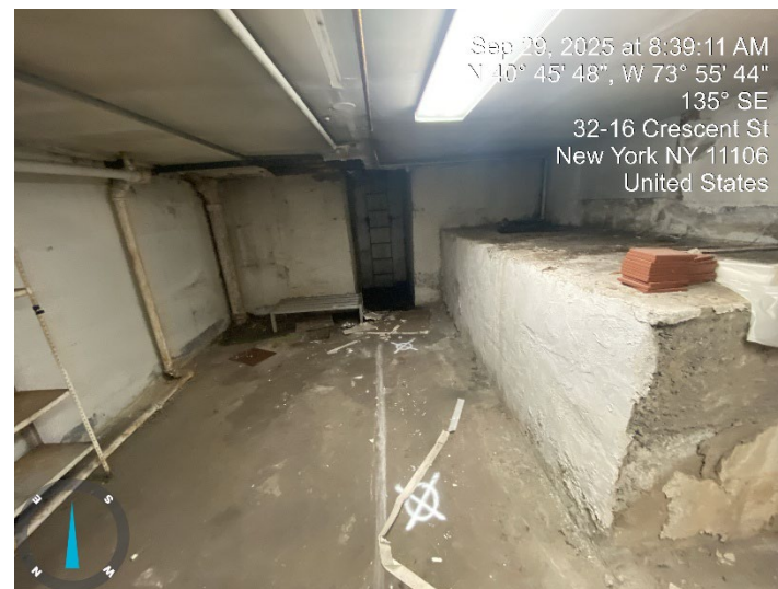
Photograph 2: Preparing to drill in one partial cellar next to the above ground storage tank, view facing south.
