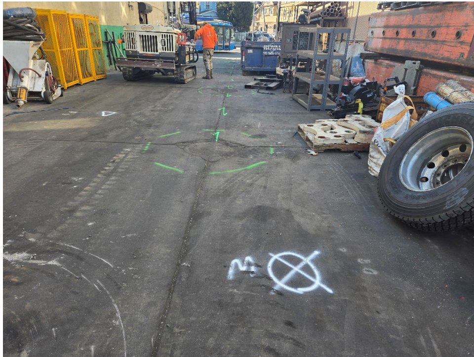
Photo 1. View of one of the cleared soil borings outside of the building on site.
