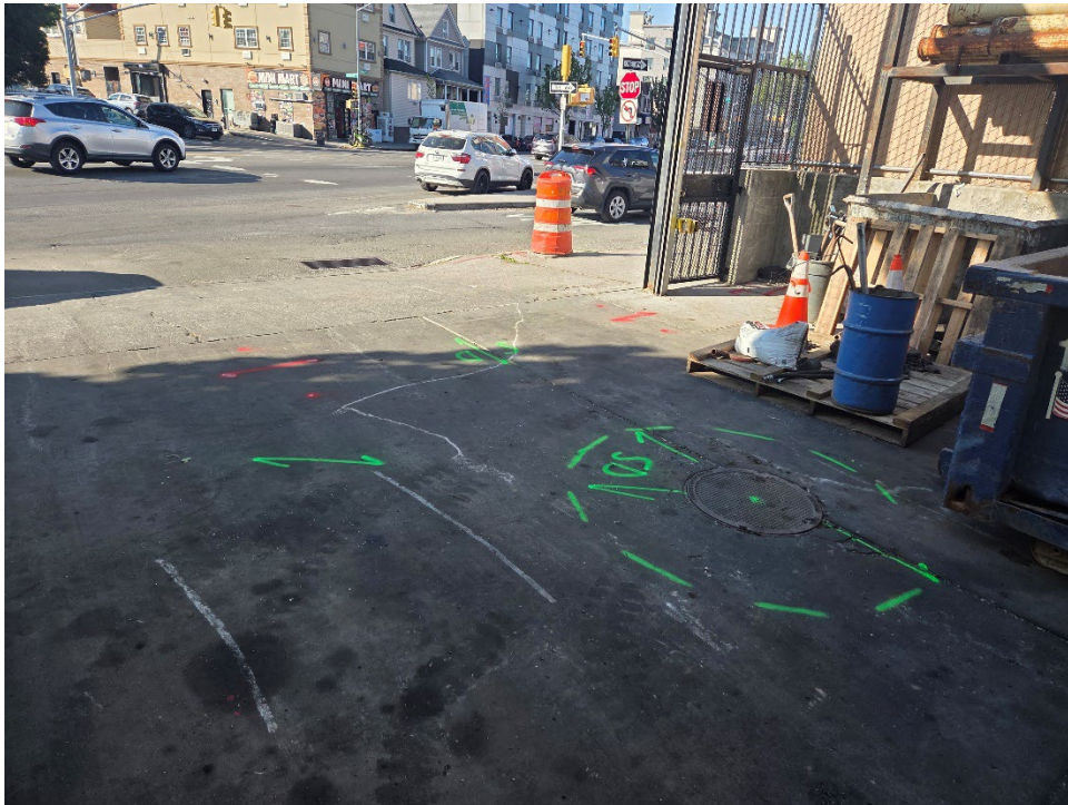
Photo 2. One of the multiple drainage structures on site.
