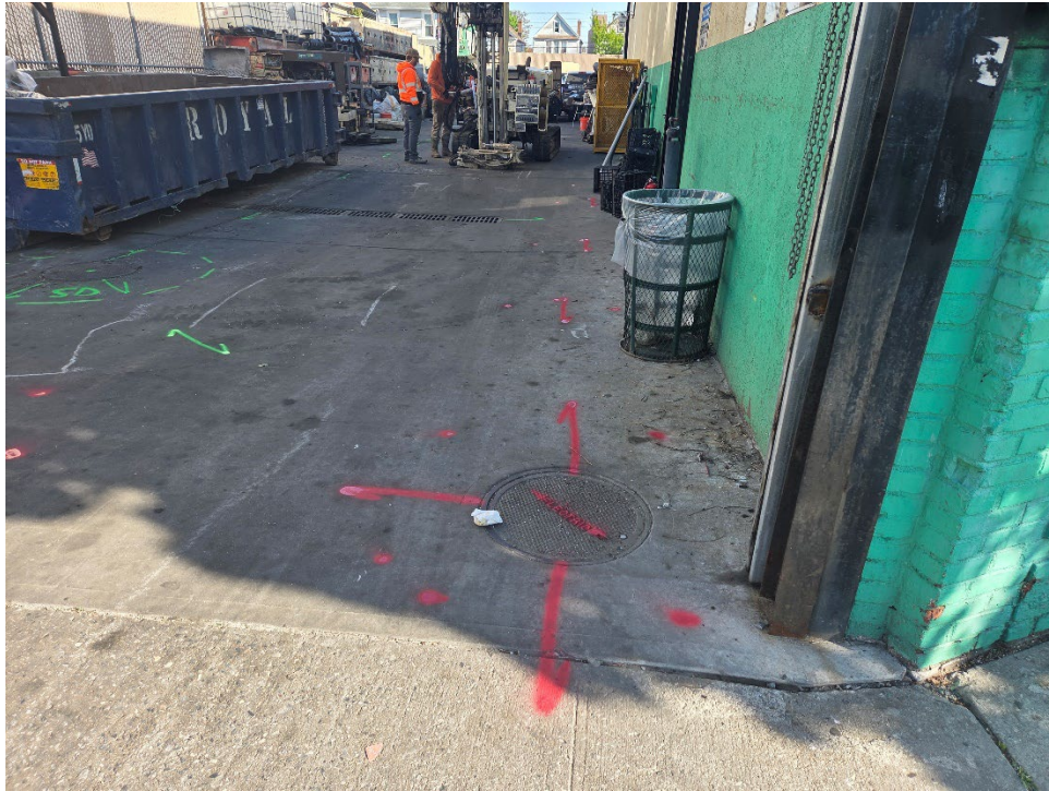
Photo 3. Drainage and electrical structures outside of the building.
