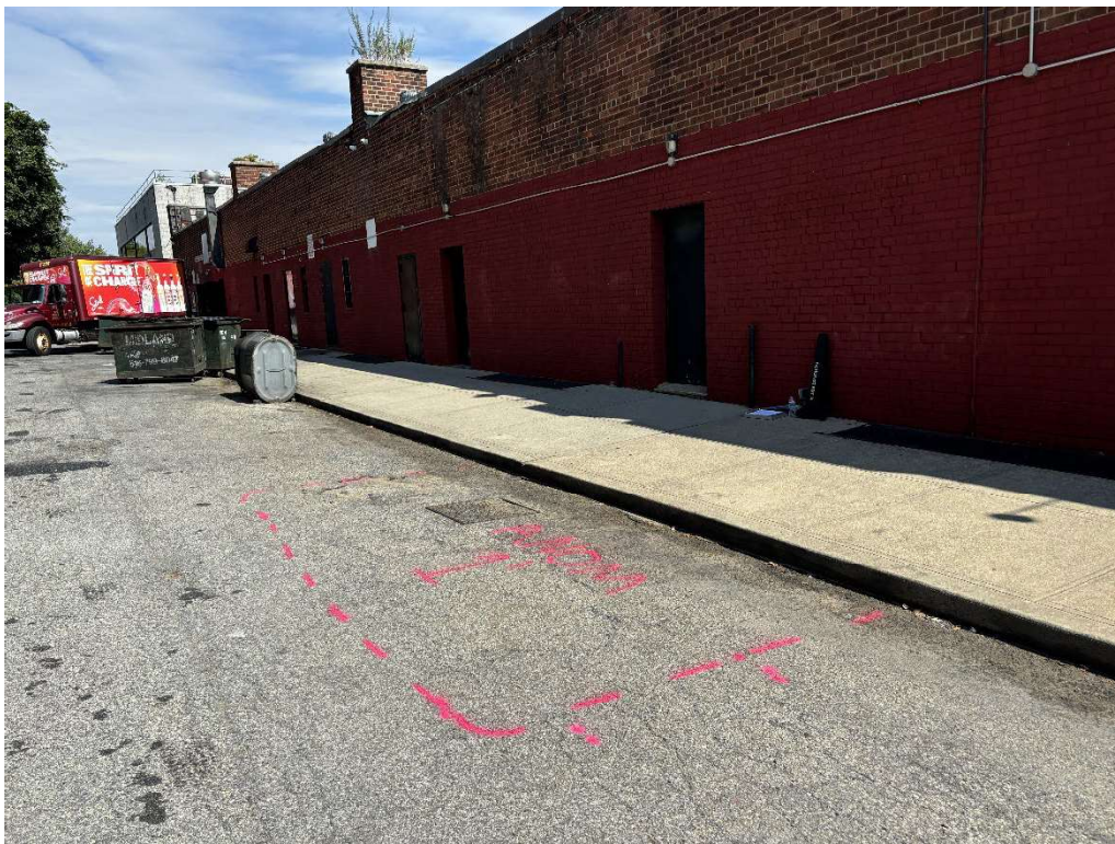
Photo 6: View of a geophysical anomaly located on the south side of the Site, behind the Webster Bank
