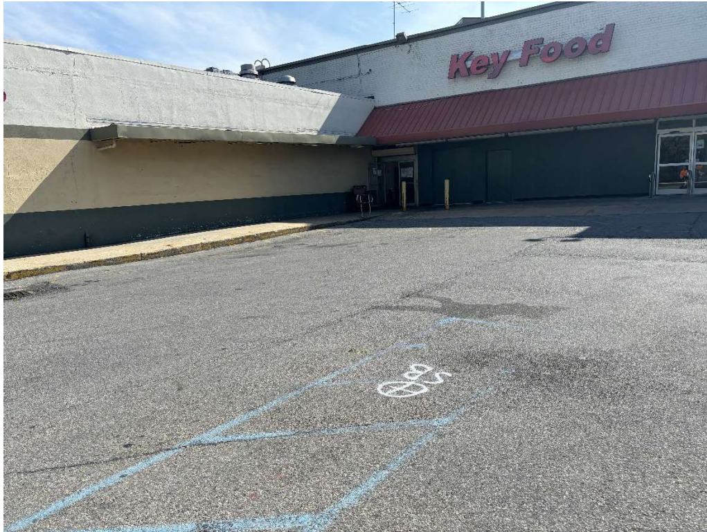
Photo 5: View of soil boring location on the west side of the Site, by Key Foods
