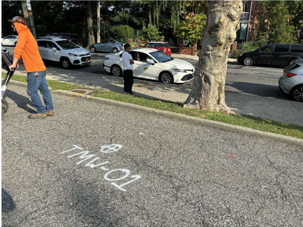
Photo 3: View of mark out for TMW-01 boring location
