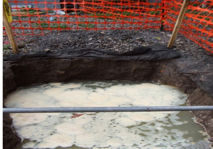
Photo 3: Groundwater in open excavation of Area 1.
