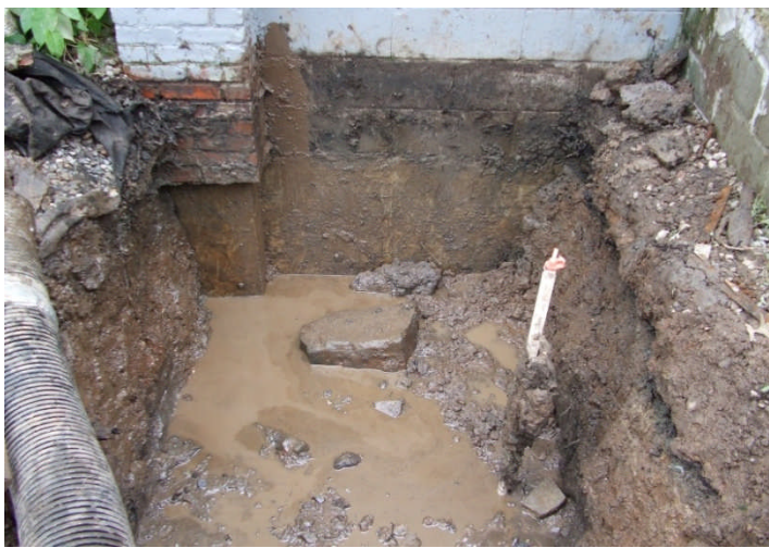
Photo 5: Exposed monitoring well MW-101S in Area 4; MW-101D was destroyed during excavation.
