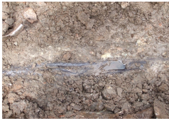
Photo 13: Broken 2-inch pipe in Area-5.
