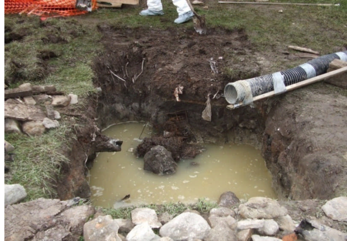
Photo 15: Preparing to dewater Area 5 at start of work day.
