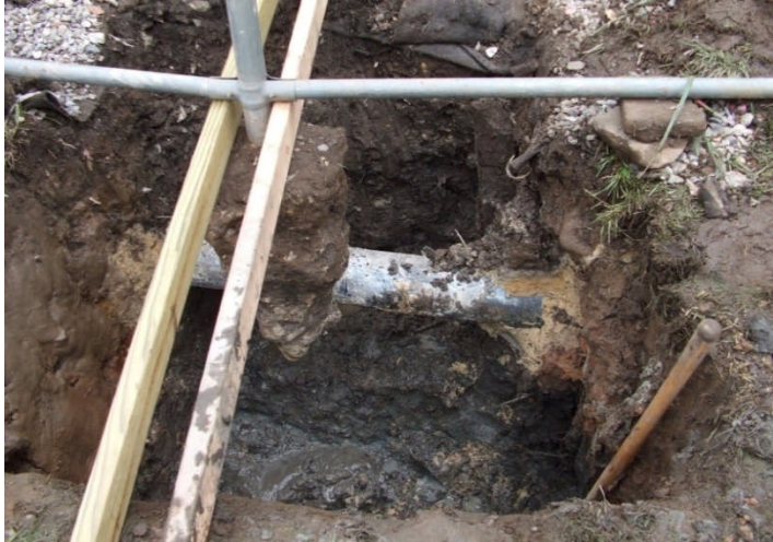
Photo 7: Exposed gas pipeline in open excavation of Area 3.
