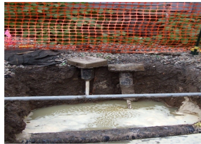
Photo 2: Gas pipeline and monitoring wells MW-102S and MW-102D exposed in open excavation of Area 2.
