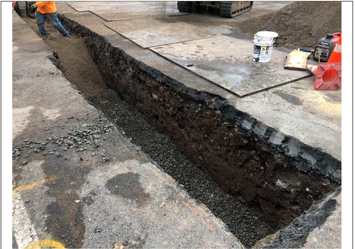
Photo 2: View of stone placed as bedding in trench.
