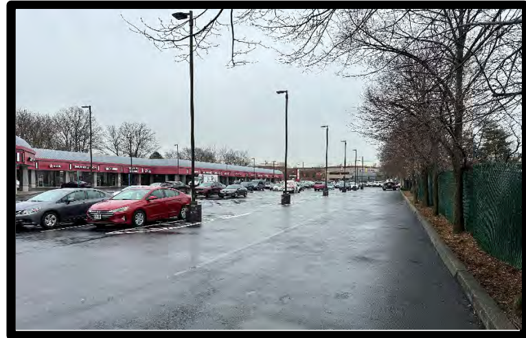
Photo 2: Parking lot looking east from far west end.
