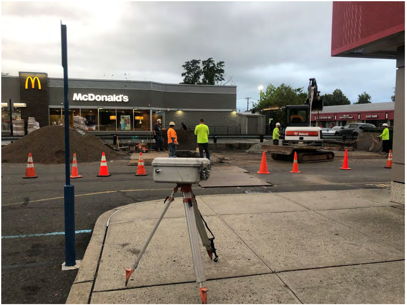
Photo 1: Looking southwest. View of CAMP station downwind of active excavation work.
