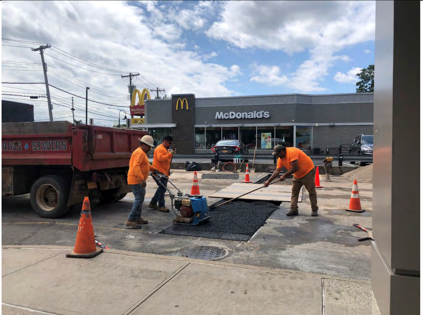
Photo 4: Looking southeast. View of Carmine placing and compacting asphalt.
