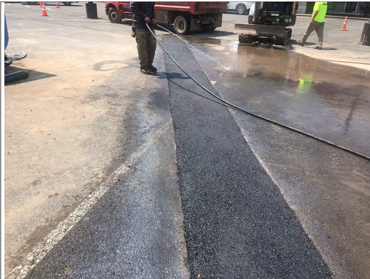
Photo 4: Looking west. View of finished work zone.
