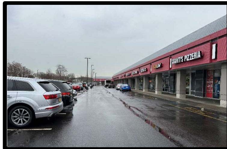
Photo 8: Front of northern building (looking west).
