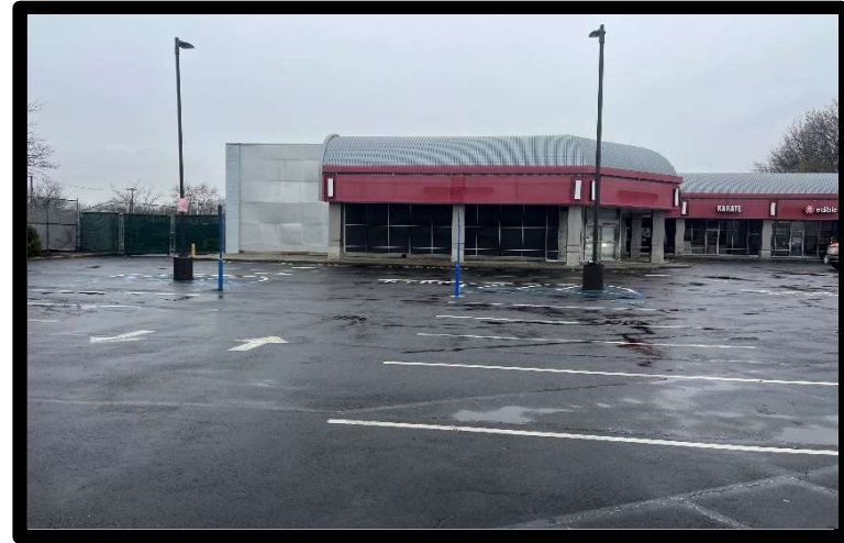
Photo 2: Parking lot looking north from far west end.
