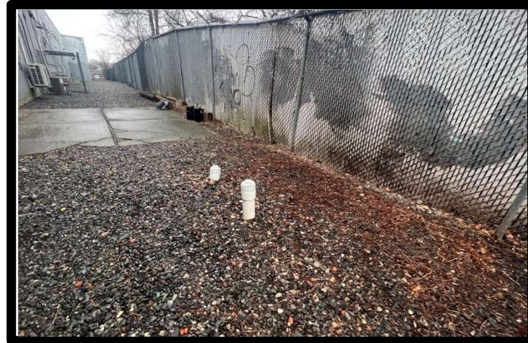
Photo 6: Gravel area in rear of northern building (west).
