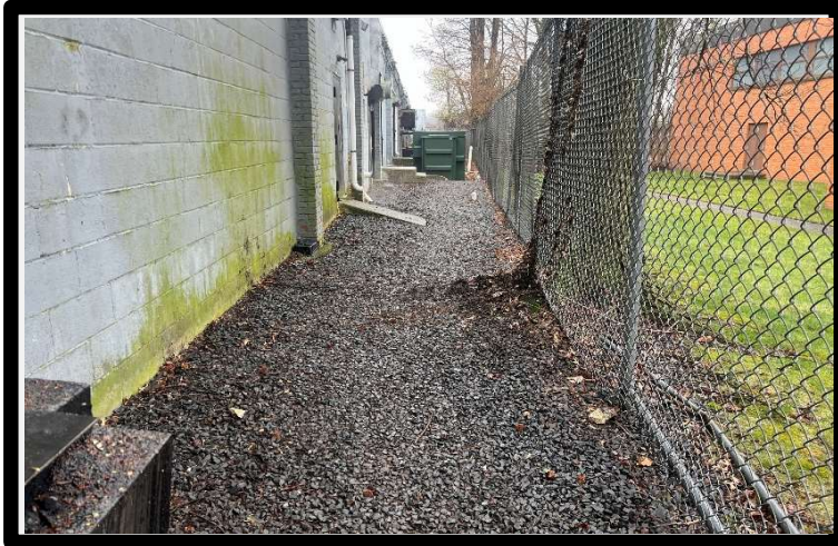
Photo 5: Gravel area in rear of northern building (east).
