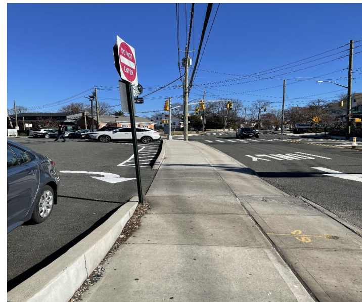
Photograph 4: View of Site Cover System and concrete sidewalk with off-Site monitoring wells looking northeast.
