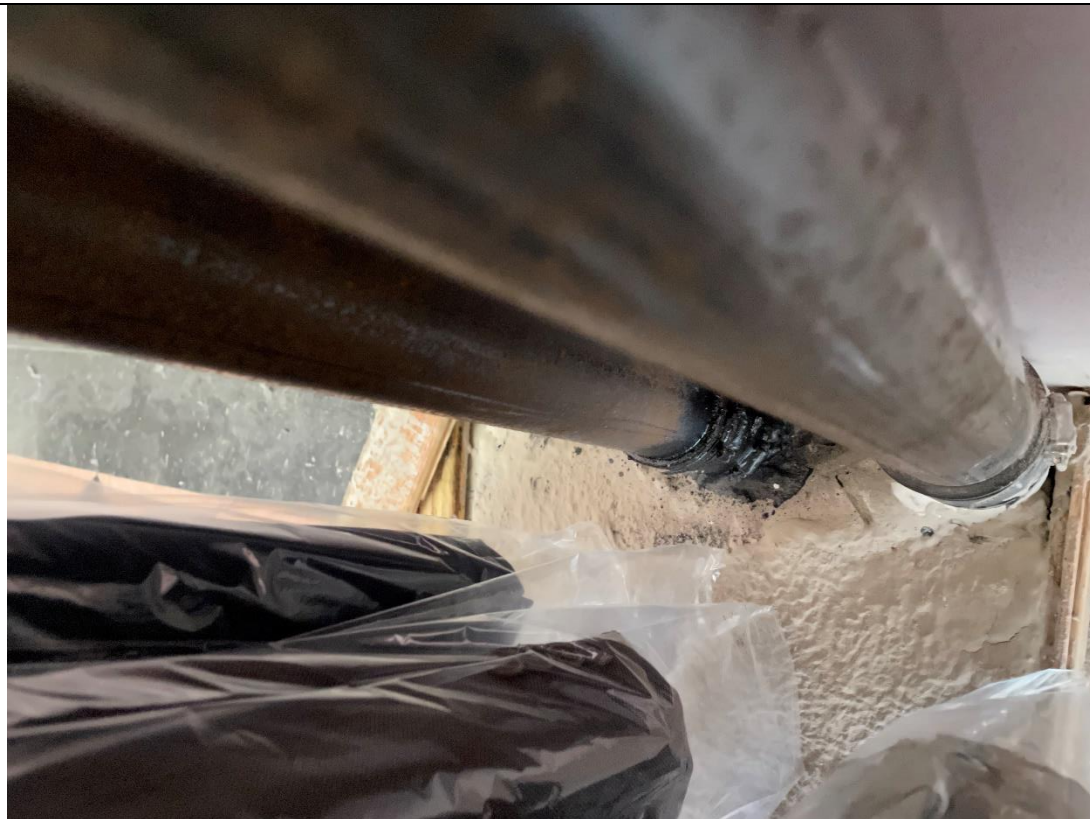
Photo 4 – From left to right, view of VEP-29 (leaking air at base of individual well-line), and VEP-17 (leaking air at trench concrete patch), facing northwest.
