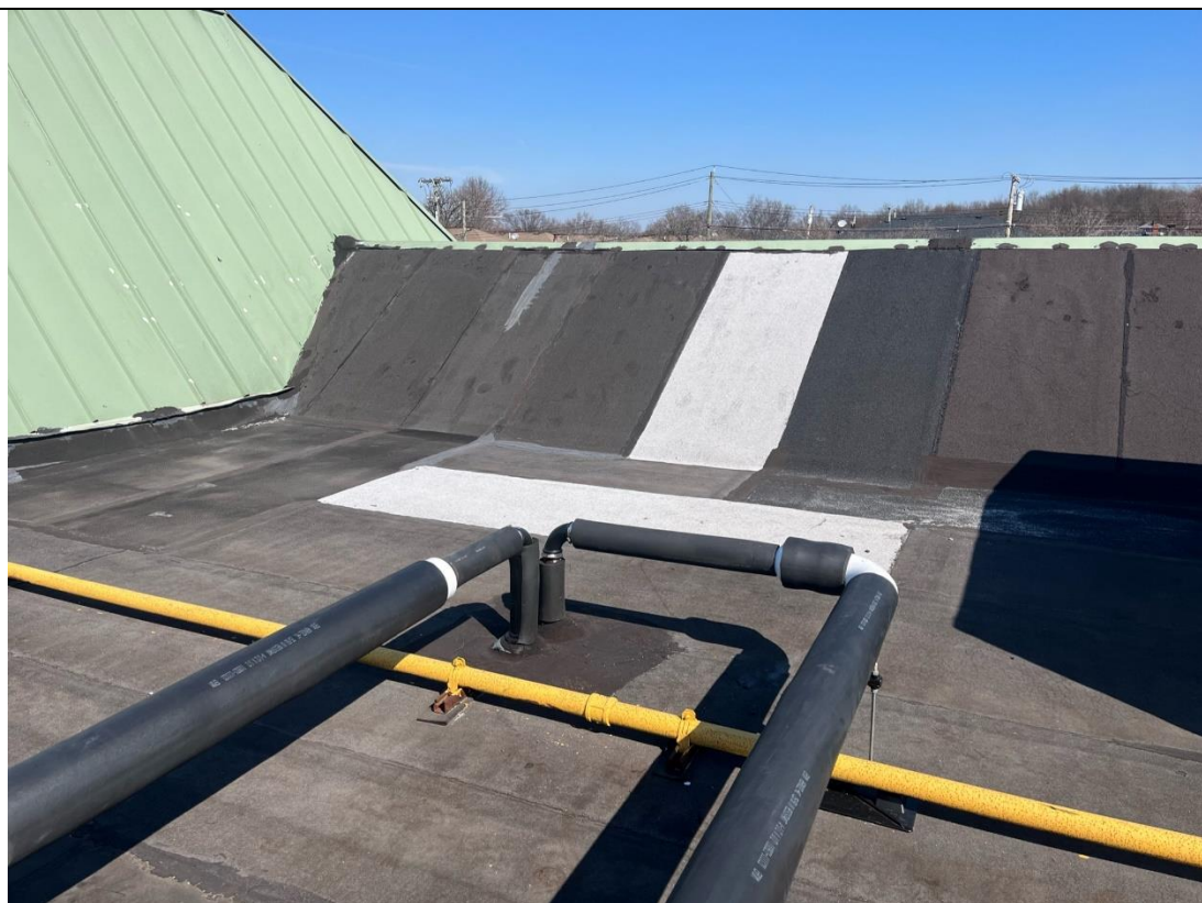
Photo 4 – View of insulated 2-inch and 4-inch sub-header piping, facing north.
