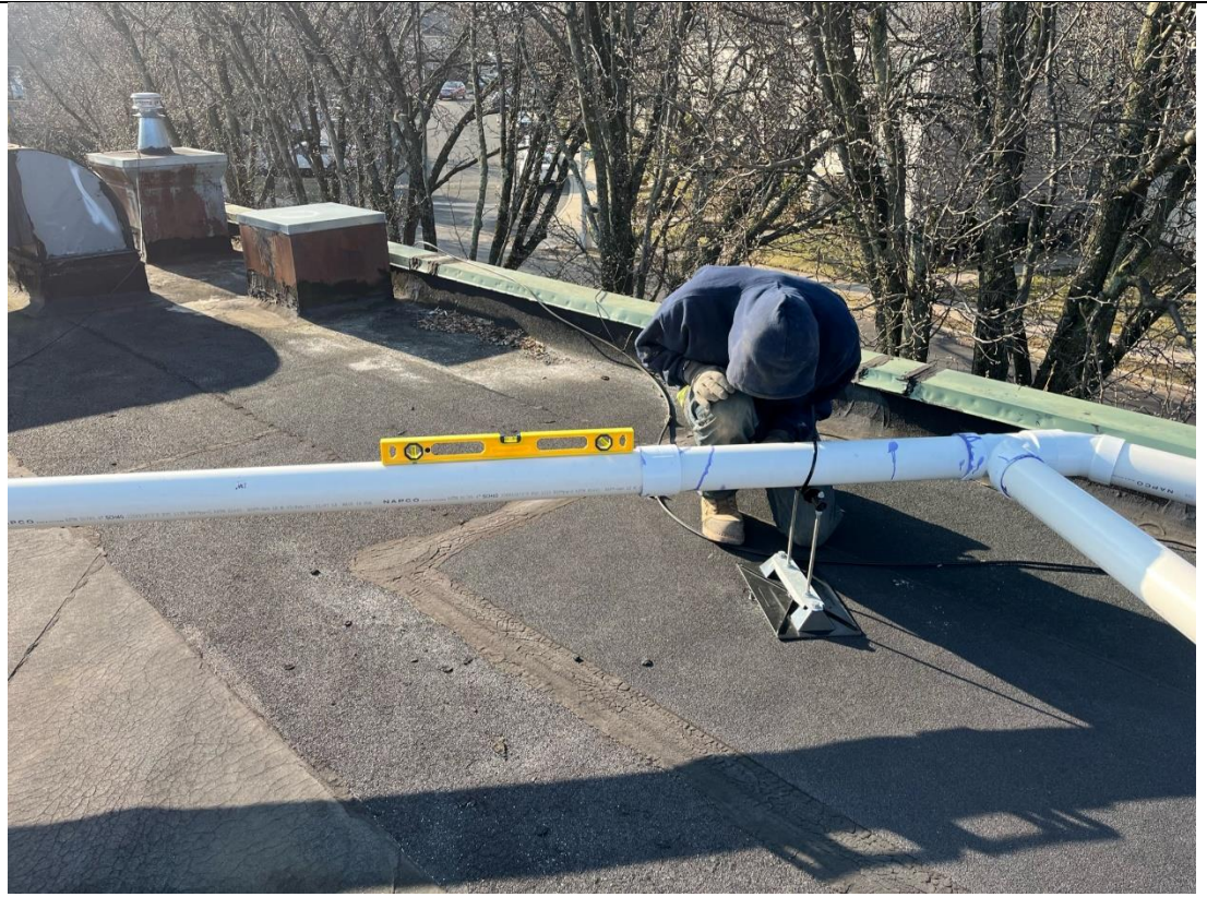
Photo 1 – View of Pennington correcting pipe sloping issues, facing south.
