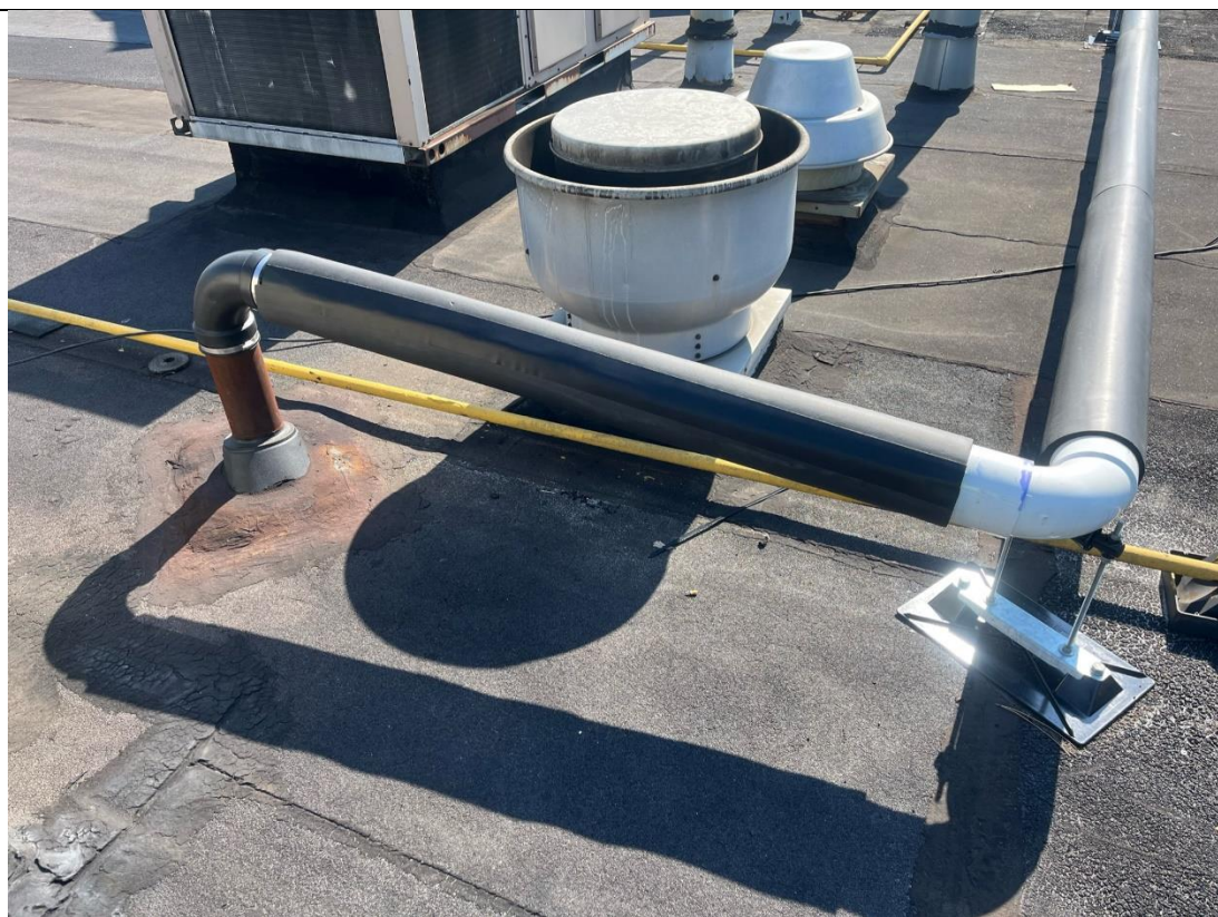
Photo 3 – View of one location where 4-inch black steel sub-header line will need to be cut down to achieve the appropriate pitch, facing southeast.
