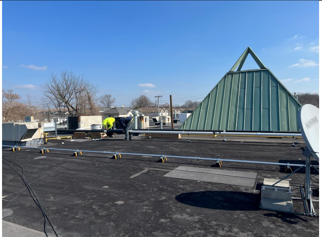
Photo 2 – View of Pennington installing insulation to 4-inch sub-header piping, facing northeast.
