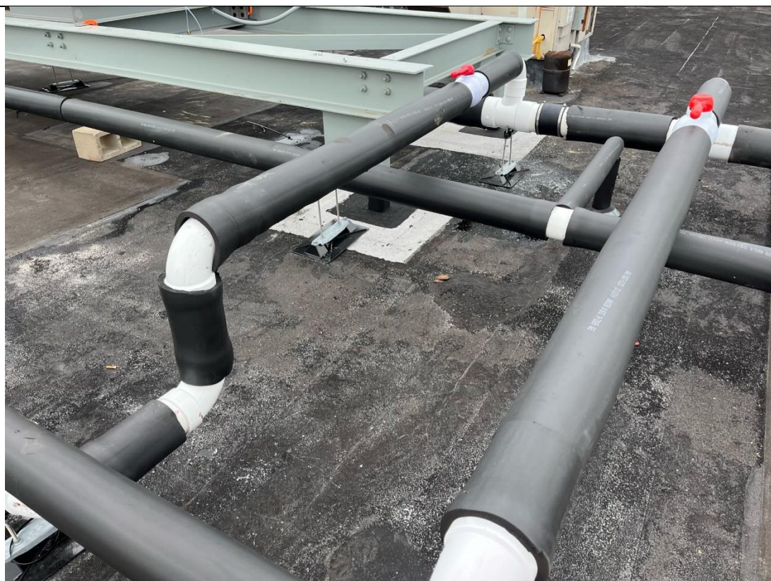
Photo 3 – View of cut and reinstalled 4-inch PVC sub-header piping, now running above nearby lines rather than below them, facing northwest.
