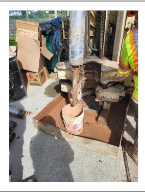
Photo 4 – ADT/Cascade grouting LMW-1B, facing north.
