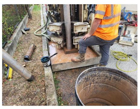
Photo 3 – ADT/Cascade removing the well casing from LMW-1A, facing north.
