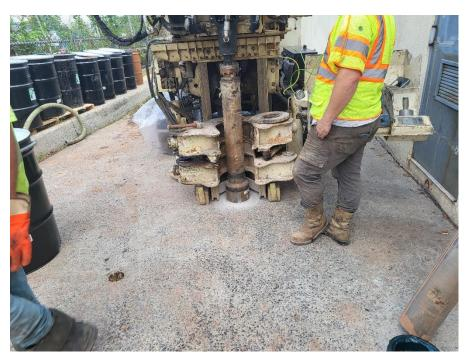
Photo 3 – ADT/Cascade removing the well casing from LMW-2, facing north.
