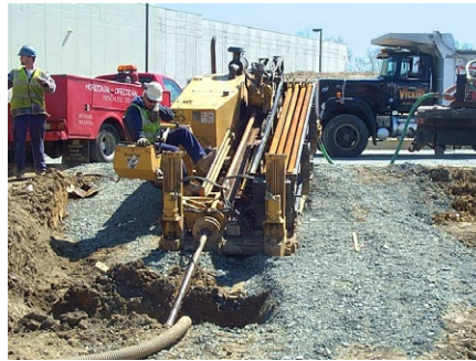
New Jersey Turnpike, Cranbury, NJ
