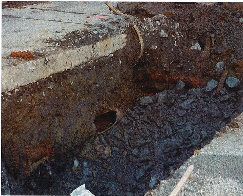
Old pipe in trench
