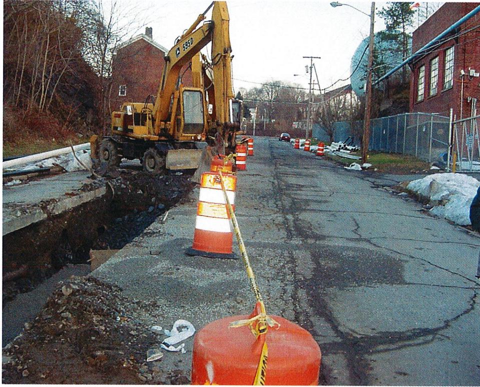
Trench for new sewer
