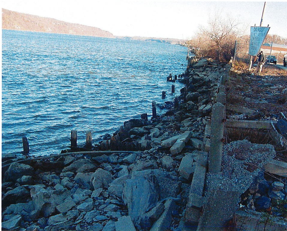
Looking north from north-central portion of site (former wooden bulkhead left of riprap)
