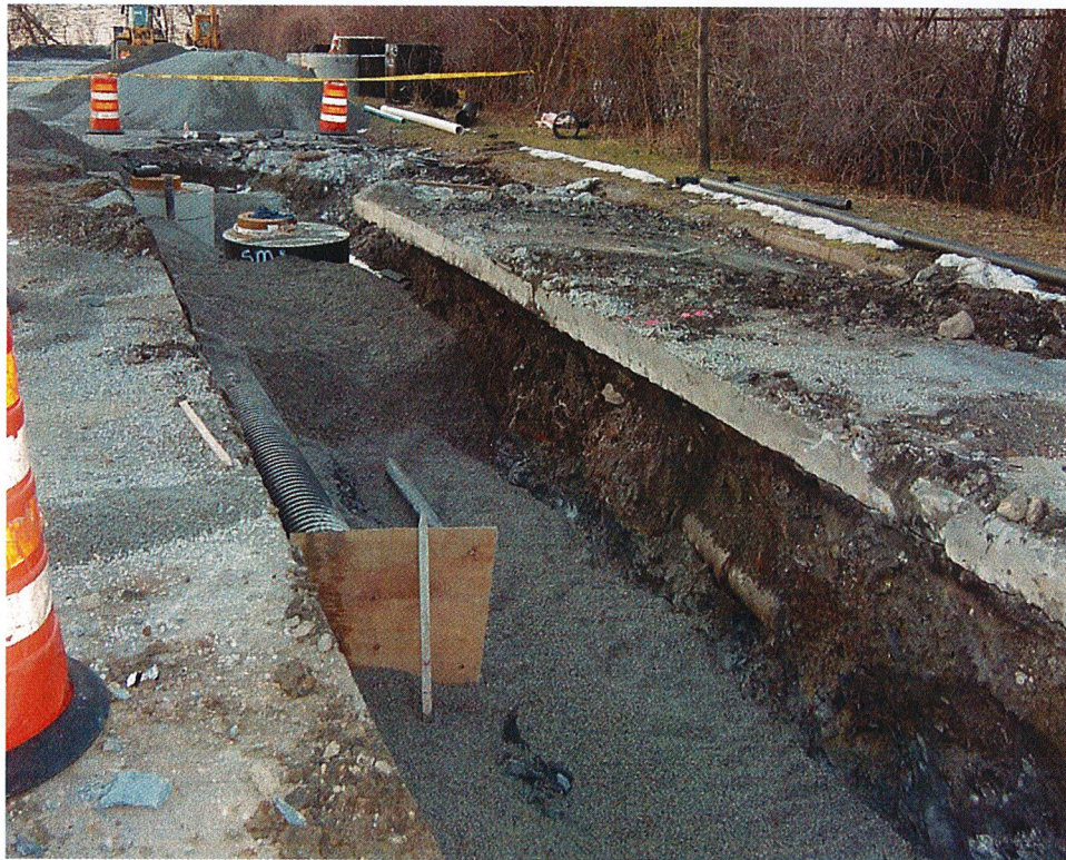
Trench for new sewer line
