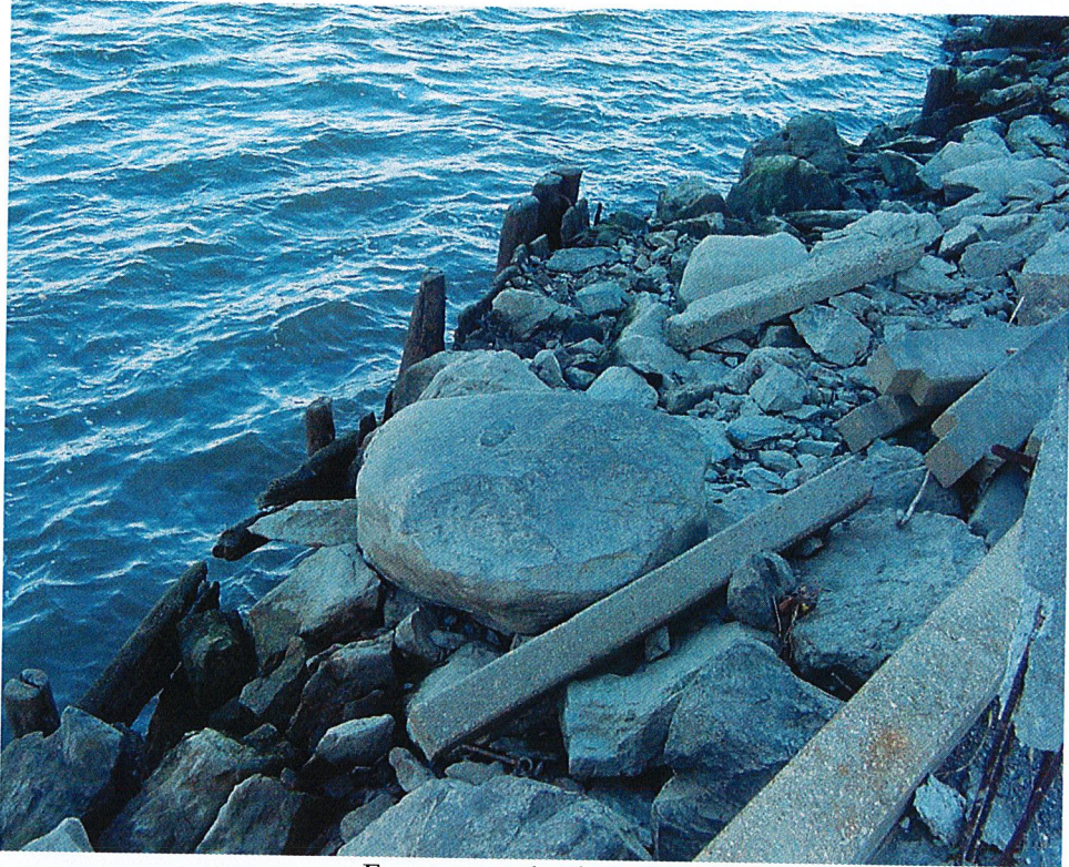
Former wooden bulkhead
