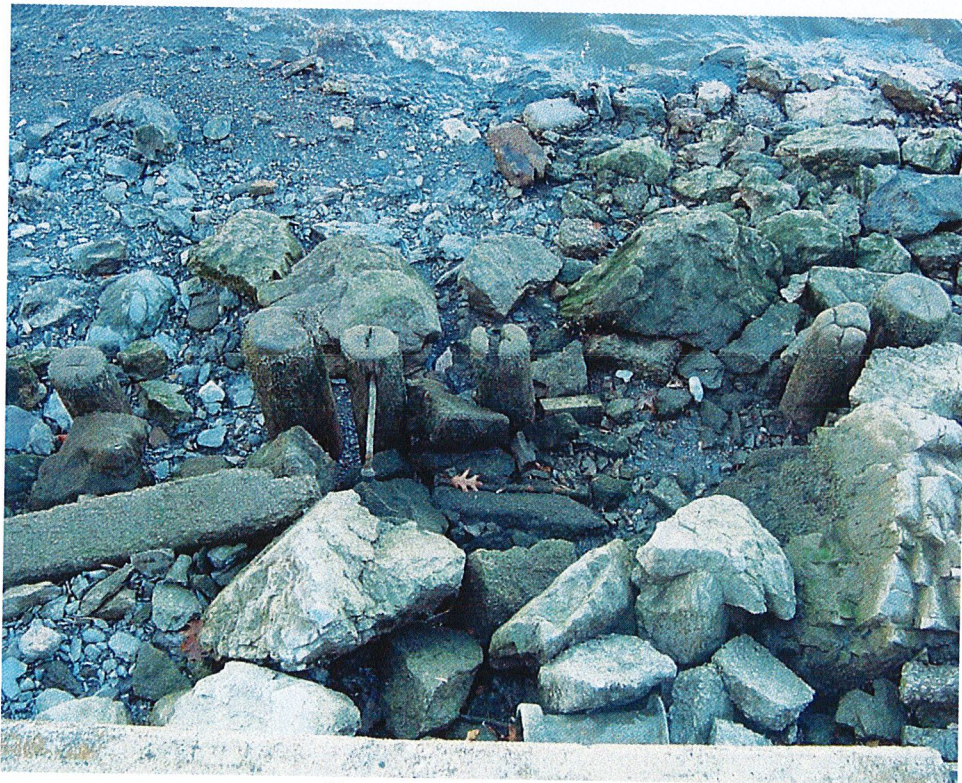
Former wooden bulkhead
