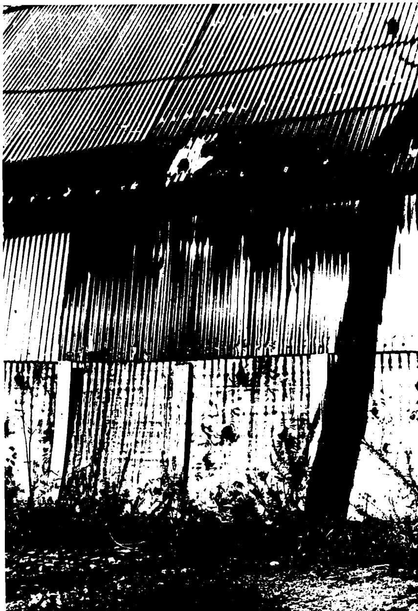
Figure III-4 - The hole in the roof of the north treatment plant (south side) is allegedly the location of an overflow vent for the storage tank. CAA solution reportedly ran out of this overflow vent and onto the ground when the operator failed to shut down the intake valve to the storage tank.
