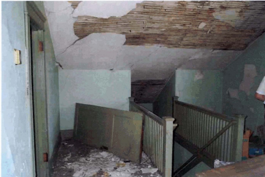
11. Deteriorated plaster, attic of main office building
