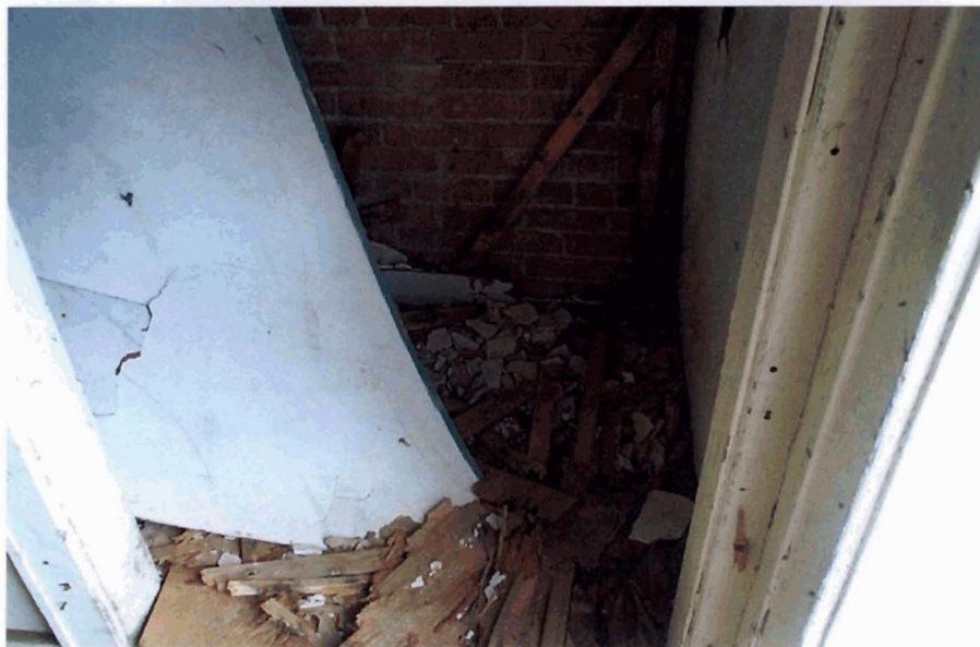
11. Deteriorated plaster, attic of main office building
