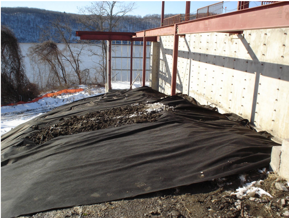
Photo 45 —Laying of geotextile demarcation barrier over the Secondary Soil Consolidation Zone (December 12, 2005)
