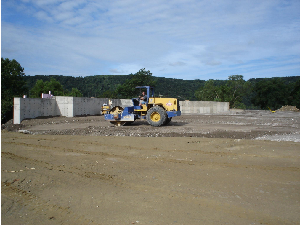
Photo 31 — Final grading and soil compacting in Primary Soil Consolidation Zone (July 28, 2005)
