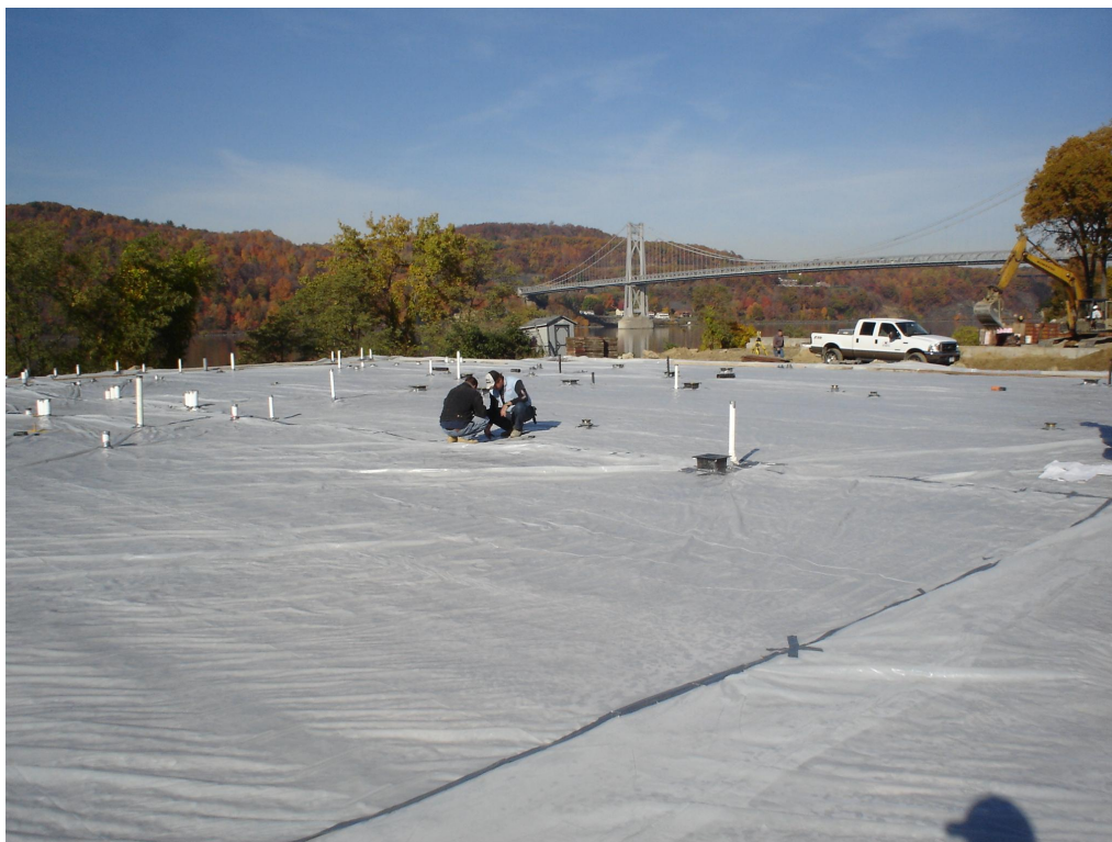
Photo 42 — View of vapor barrier over coarse aggregate (November 4, 2005)
