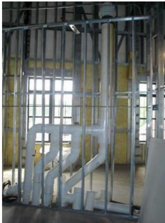
Photo 50 — Sub-slab venting system piping at manifold and inline centrifugal fan (June 20, 2006)
