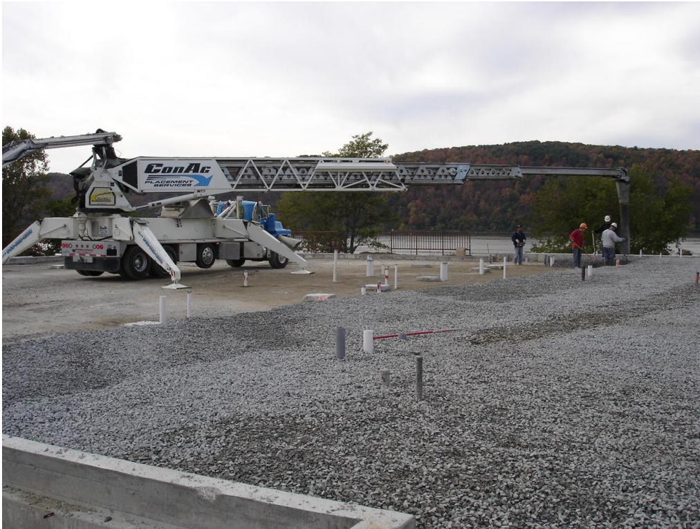
Photo 39 — Installation of stone for sub-slab venting system (October 2005)
