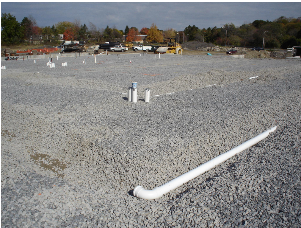
Photo 40 — View of sub-slab venting system piping looking northeast (October 28, 2005)
