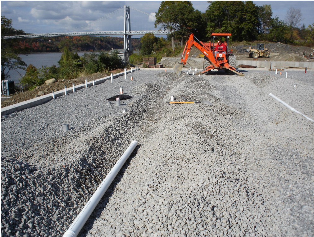
Photo 41 — View of sub-slab venting system piping looking northeast (October 28, 2005)
