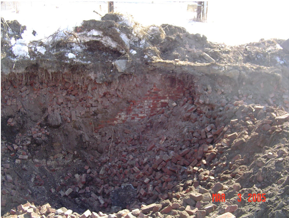
Photo 14 — Brick and building demolition debris excavated in the northeast soil mound area (March 3, 2005)
