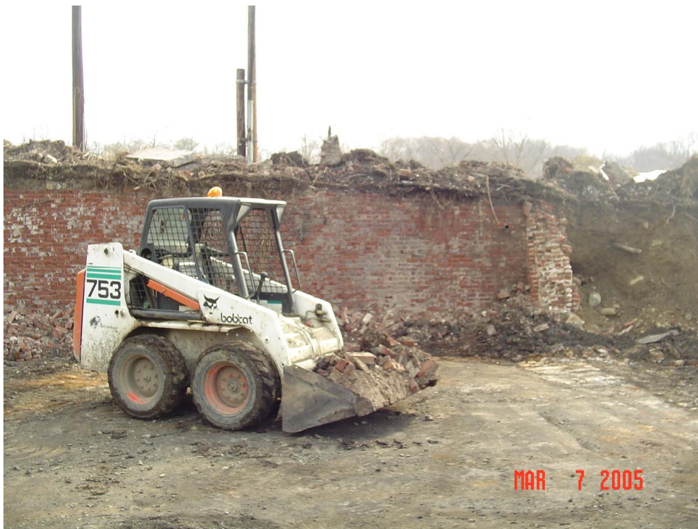
Photo 19 — Excavating residual soil on top of basement floor encountered in the northeast soil mound area (March 7, 2005)
