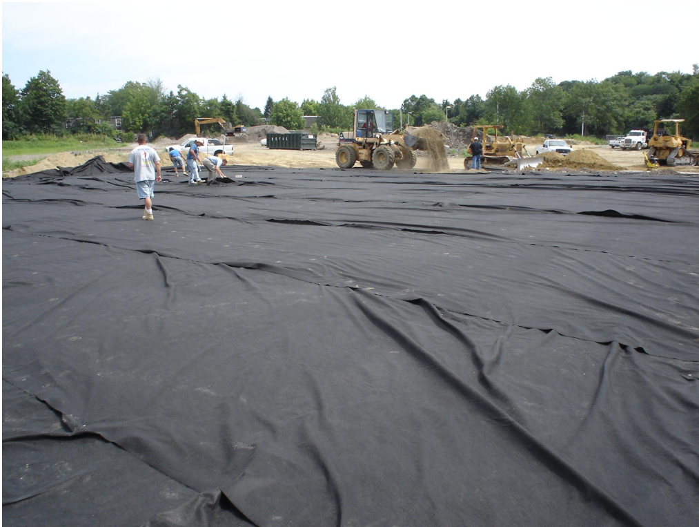
Photo 32 — Geotextile demarcation layer over the Primary Soil Consolidation Zone (July 28, 2005)
