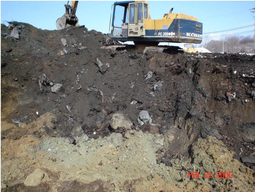
Photo 5 — Excavation of soil mixed with trash bags full of leaves in the southern landfill area (February 22, 2005)
