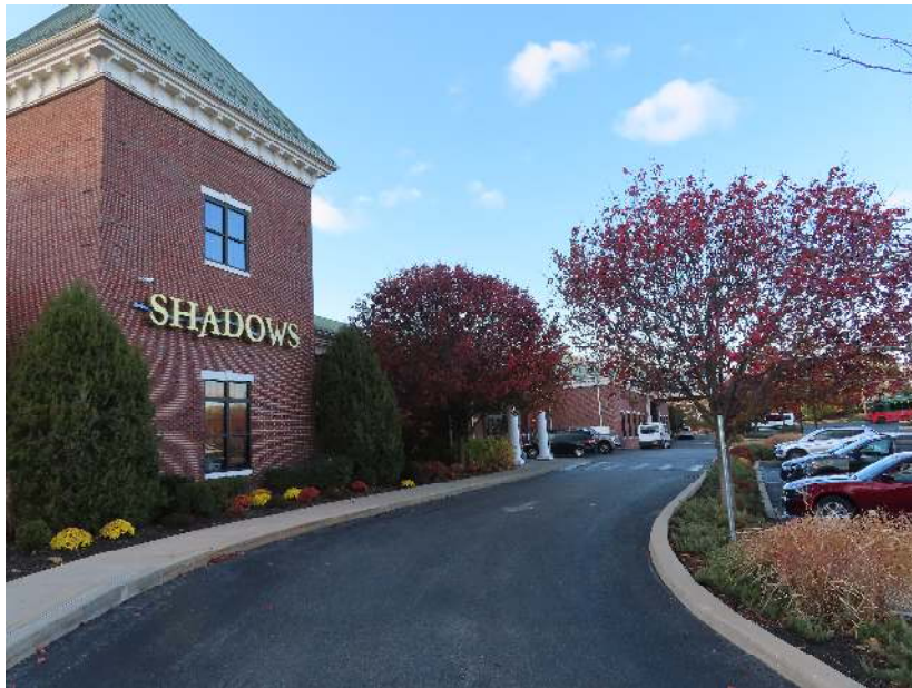
Photo 2: Front portion of facilities.
