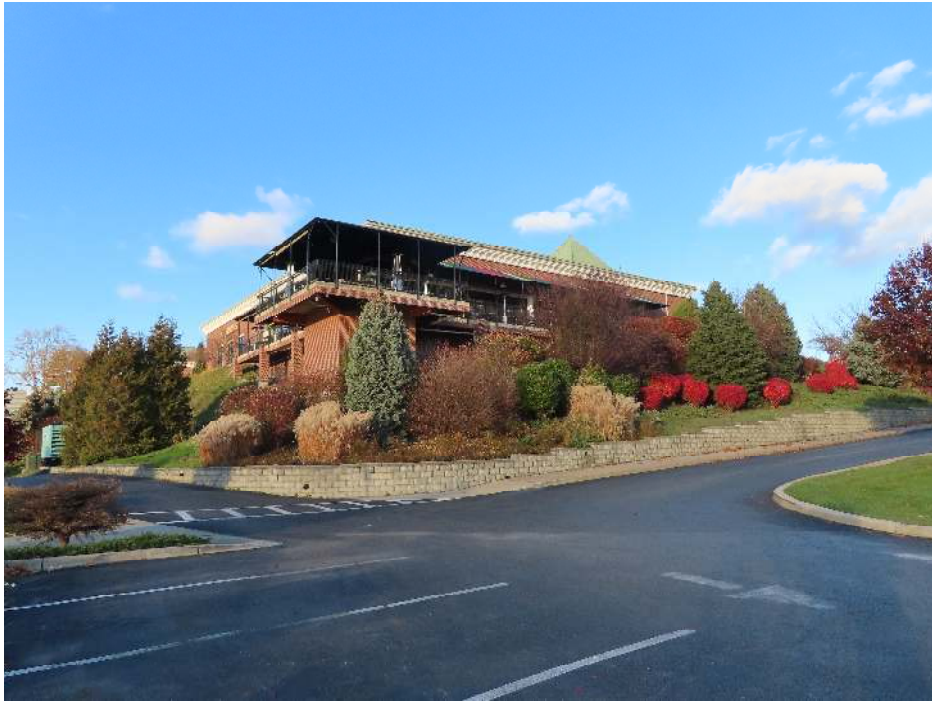
Photo 1: Area of consolidation Zone to south of building
