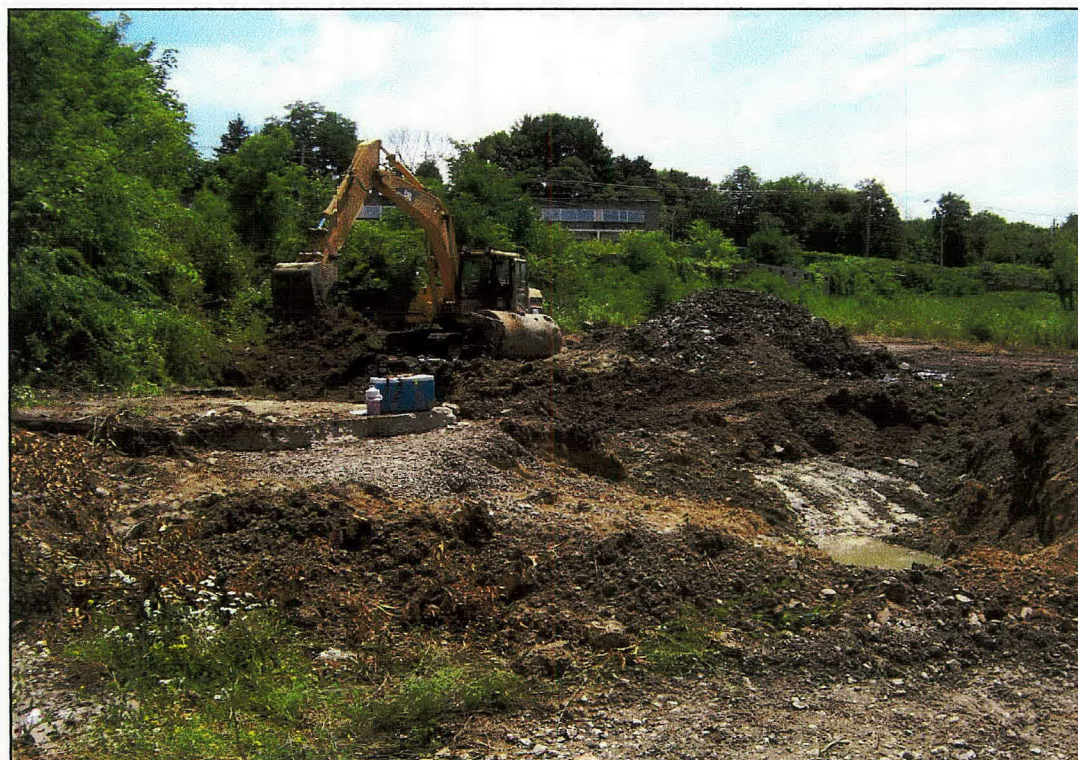
Photo 6: A view of the extents of the excavation. The easternmost portion is being backfilled.
