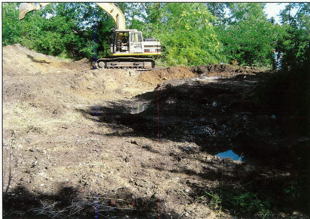
Photo 2: Non-impacted surficial soil cleared from the excavation area.
