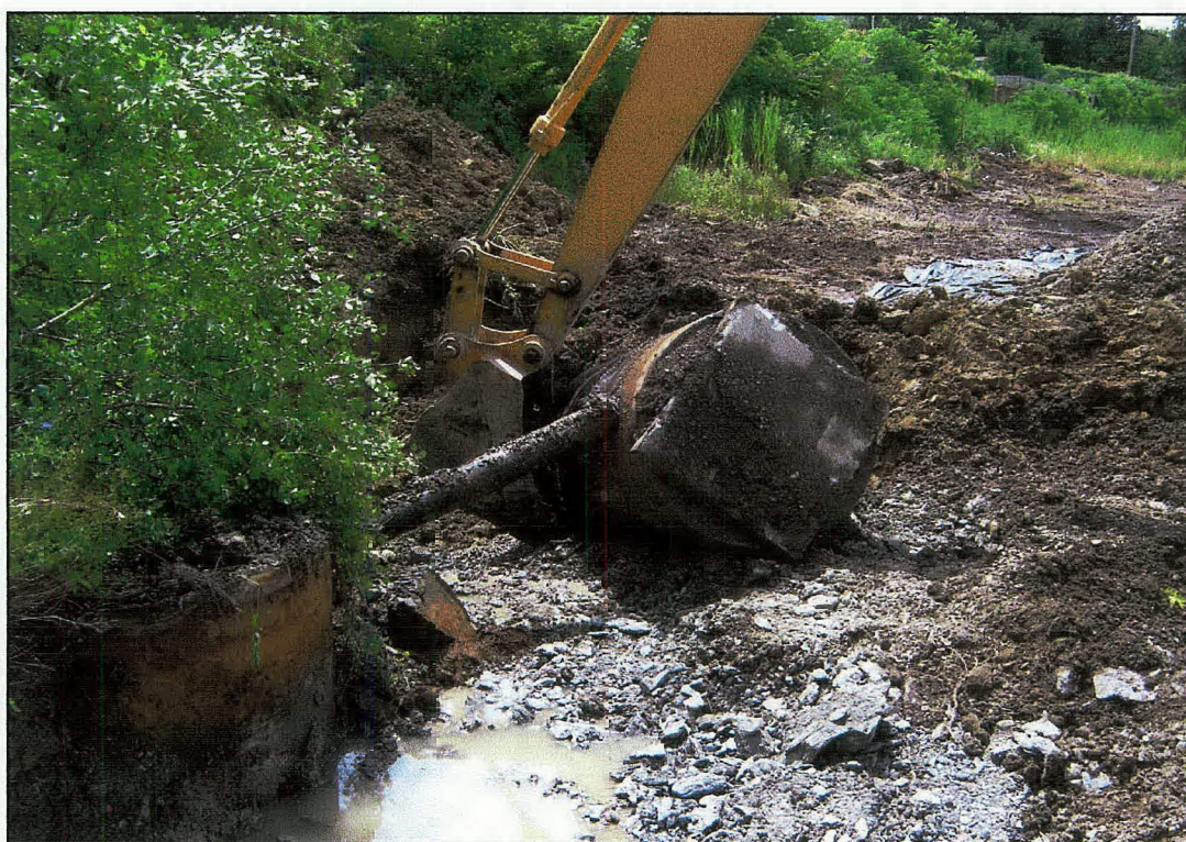
Photo 4: Removal of the likely source of impacts – assumed to be a field-fabricated oil/water separator.
