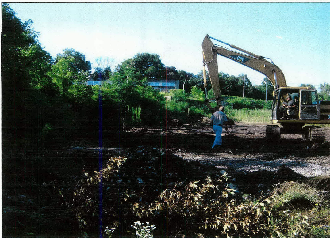
Photo 1: Area cleared by Volunteer prior to soil excavation work.
