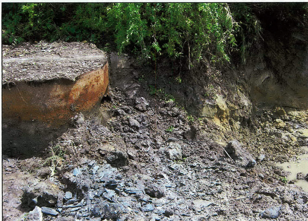
Photo 5: A view of the northern tank and the excavation where the southern tank formerly sat. The clay confining material can be seen in the background and shale bedrock in the foreground.
