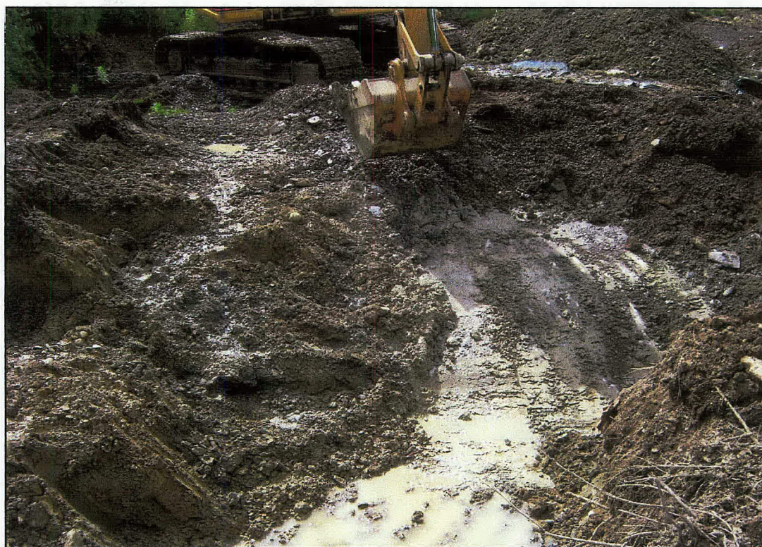
Photo 3: Bedrock scraped clean at the western portion of the excavation.
