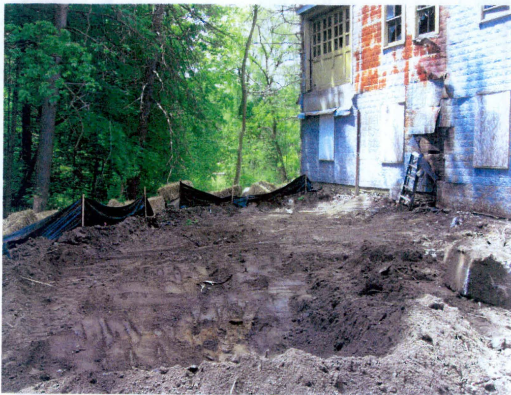
Surface soil removal on eastern side of building. View to the south. 5-15-08.
