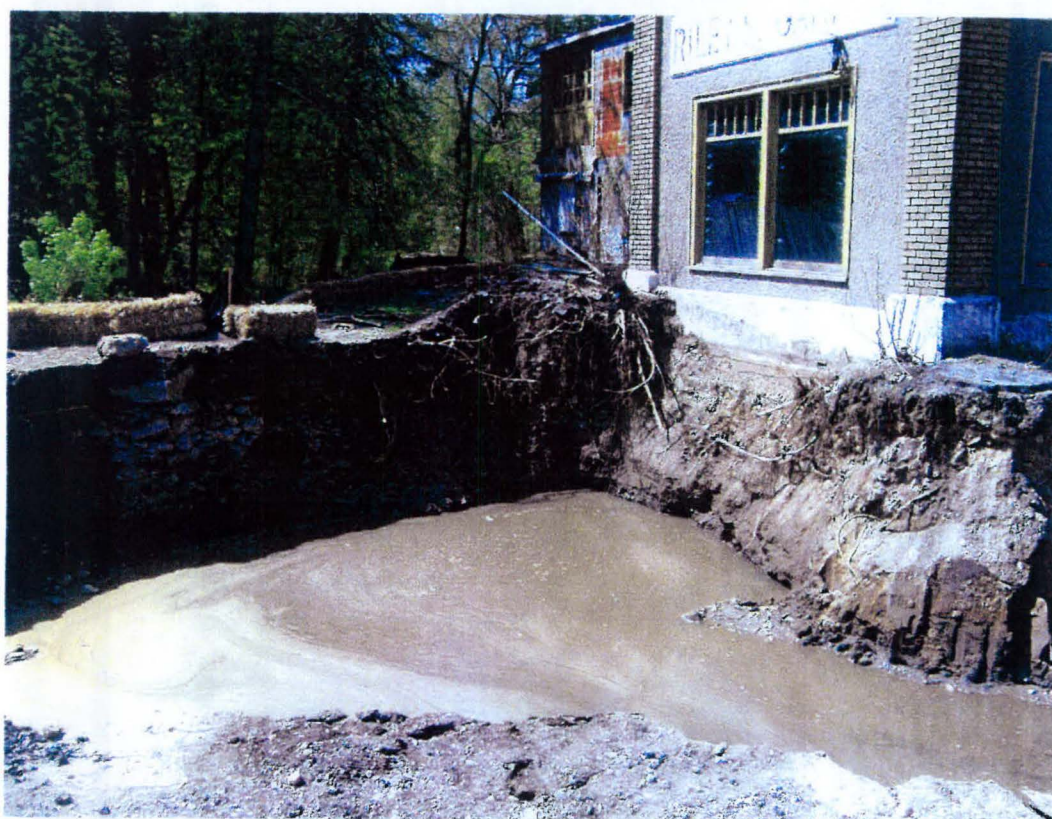
Gasoline part of completed combined gasoline UST and pump island excavation. View to the southwest. 5-1-08.
