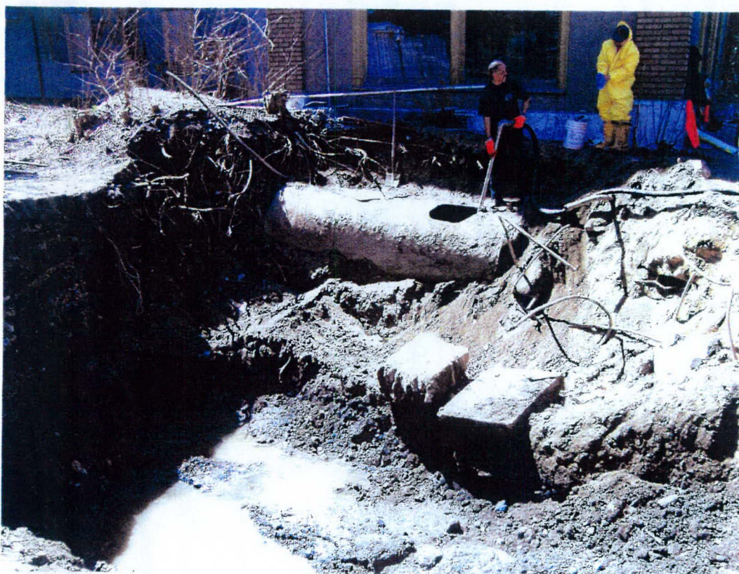
1,000-gallon gasoline tank, Tank #4. View to the northeast. 4-17-08.
