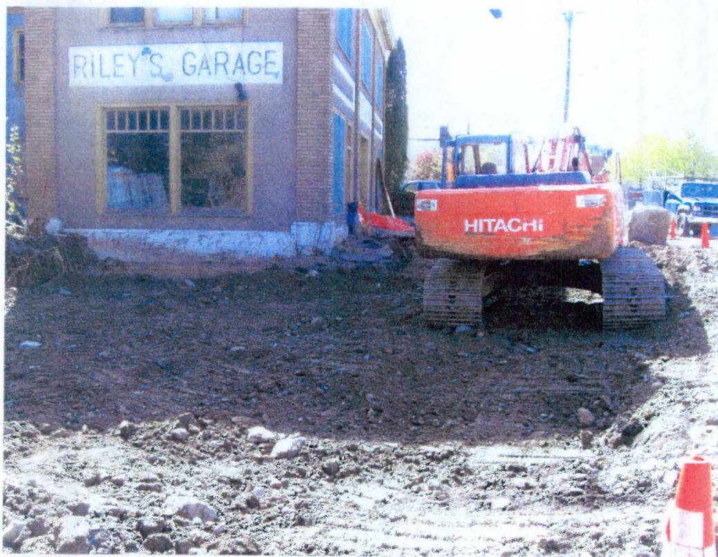
Backfilling partially completed for combined gasoline UST and pump island excavation. View to the northeast. 5-2-08.
