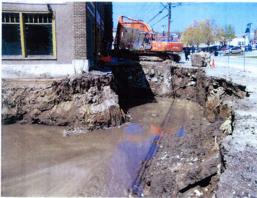
Completed combined gasoline UST and pump island excavation. View to the northeast. Pump island excavation in background; gasoline UST excavation in foreground. 5-1-08.
