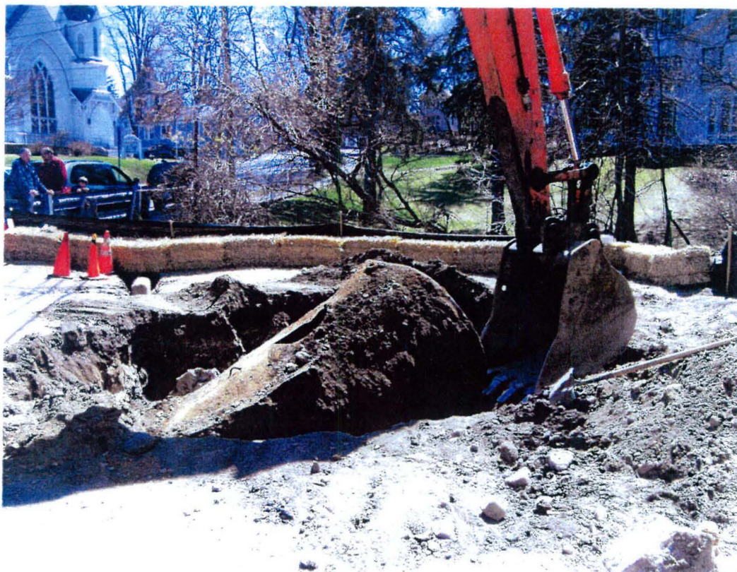
Removal of 2,000-gallon gasoline tank, Tank #2. View to the southeast. 4-16-08.
