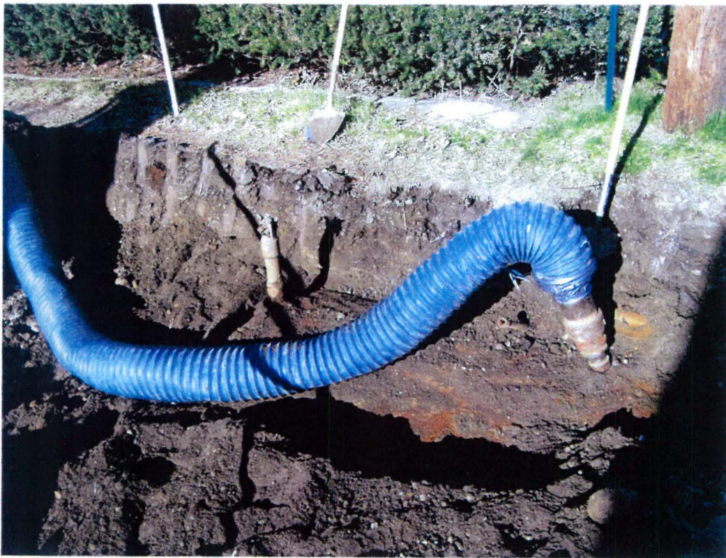
Removal of liquid from 550-gallon waste oil tank, Tank #1. View to the west. 4-16-08.
