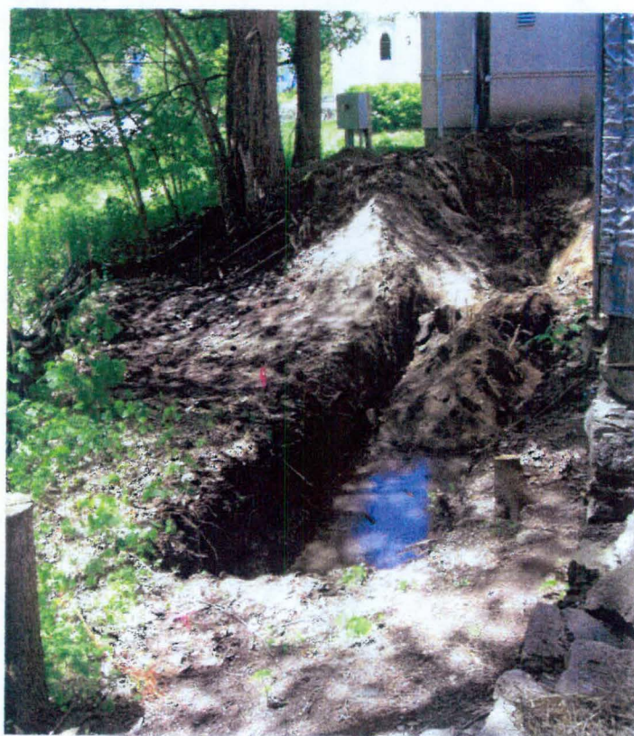
Completed floor drain outfall excavation. View to the west. On-site building to the right. 5-14-08.
