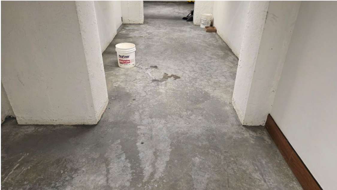
Photograph #14: View of the hallway section in the west basement. (01-22-2026)
