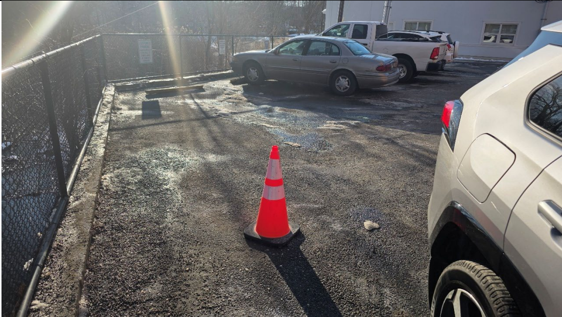
Photograph #3: Facing southwest, view of the parking lot located south of the building. (01-22-2026)
