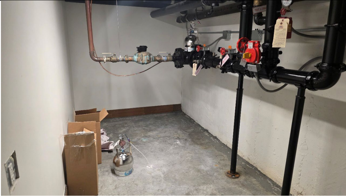
Photograph #13: View of the northern section in the west basement. (01-22-2026)
