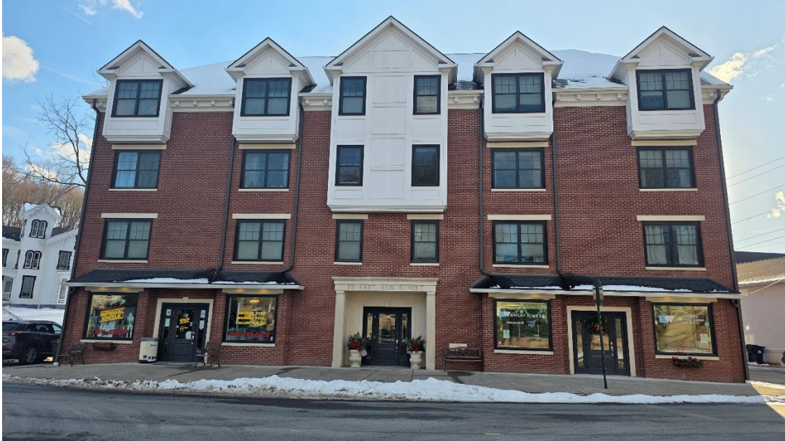
Photograph #1: Facing south, view of the main entrance to the building located on the subject property. (01-22-2026)
