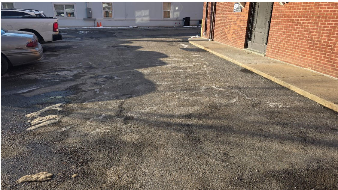
Photograph #4: Facing west, view of the parking lot/southern exterior located south of the building. (01-22-2026)
