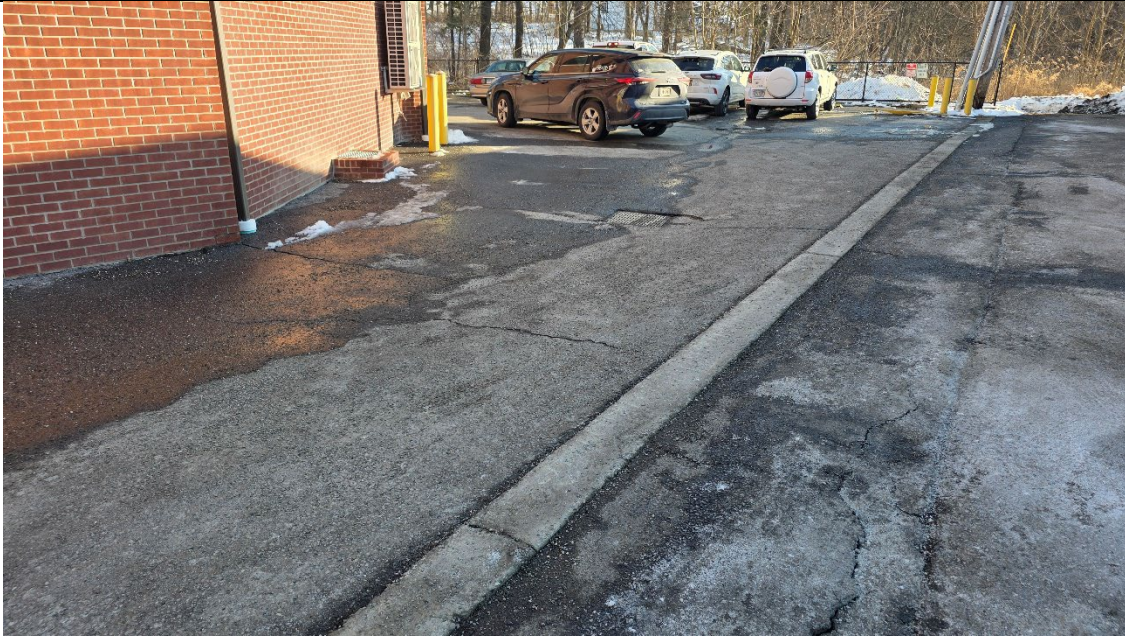
Photograph #7: Facing south, view of the western exterior of the building. (01-22-2026)
