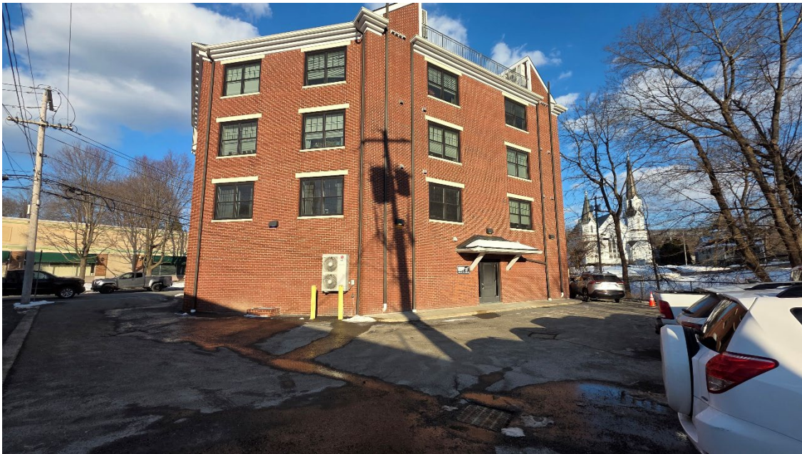
Photograph #6: Facing north, view of the parking lot/southern exterior located south of the building. (01-22-2026)
