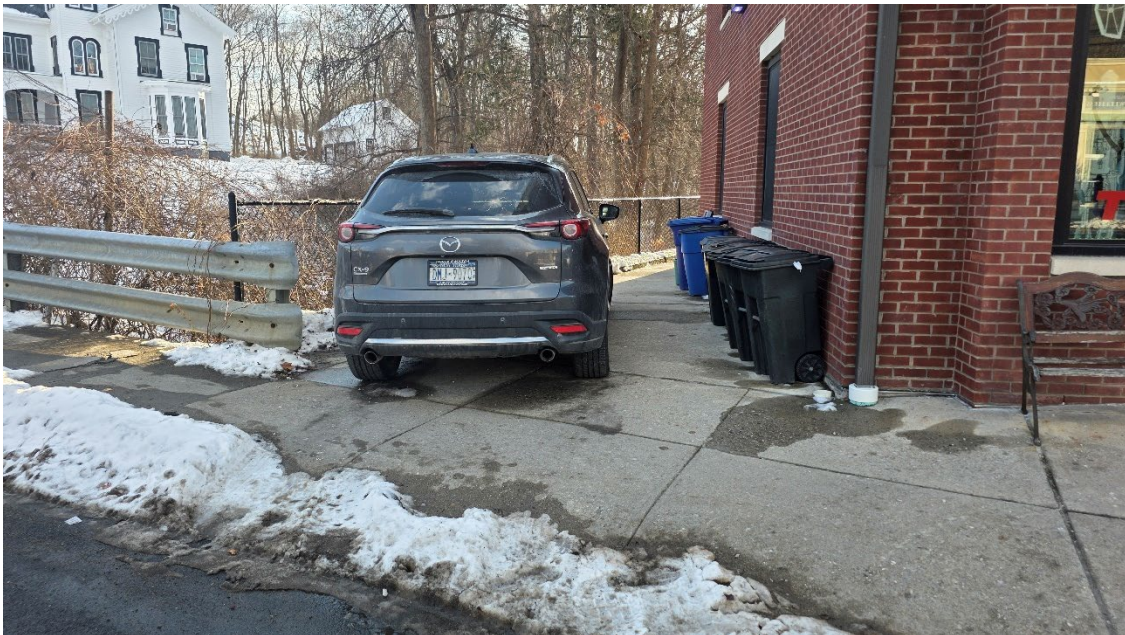
Photograph #2: Facing south, view of the eastern exterior of the building. (01-22-2026)
