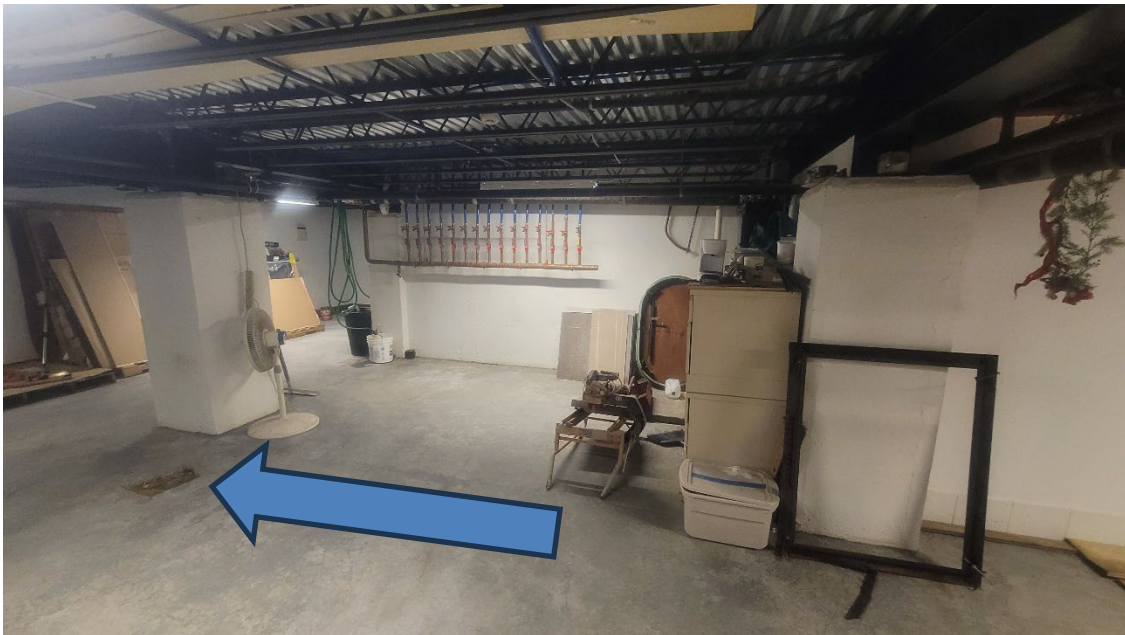
Photograph #12: View of the interior of the west basement and view of the cut-out concrete square section. (01-22-2026)
