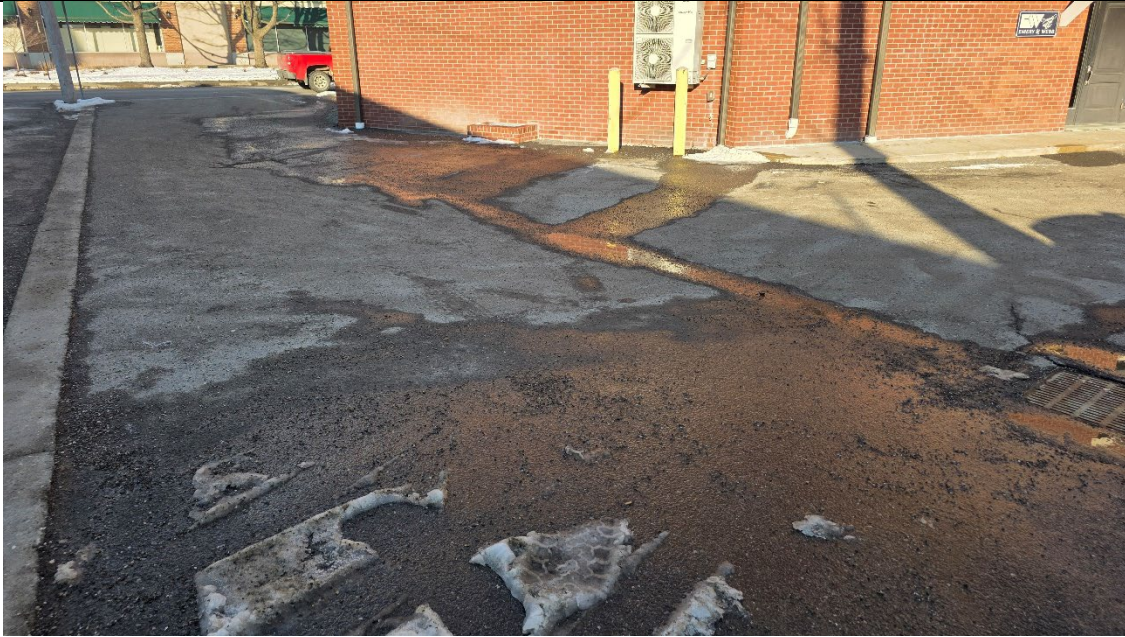
Photograph #5: Facing north, view of the parking lot/southern exterior located south of the building. (01-22-2026)
