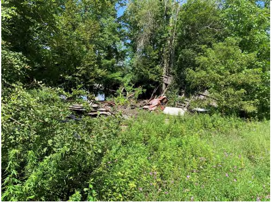
Photo 1 – Auto Garage East (Collapsed).
