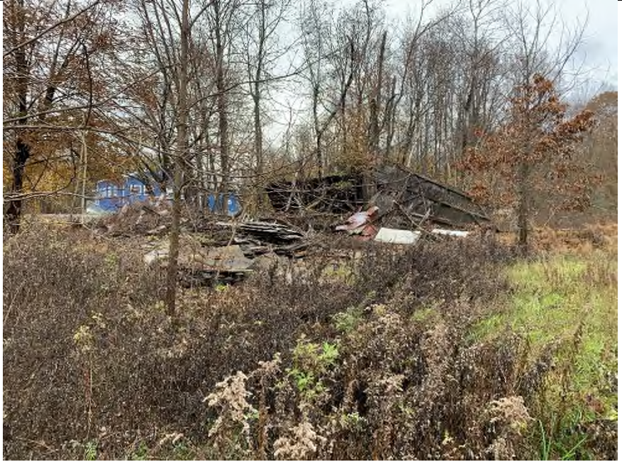
Photo 1 – Auto Garage East (Collapsed).
