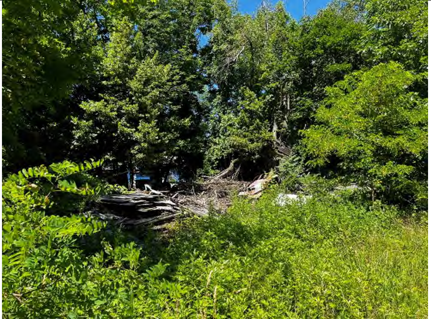
Photo 1 – Auto Garage East (Collapsed).
