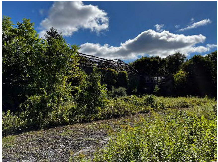
Photo 16 – Brookside structure, severe deterioration of roof.
