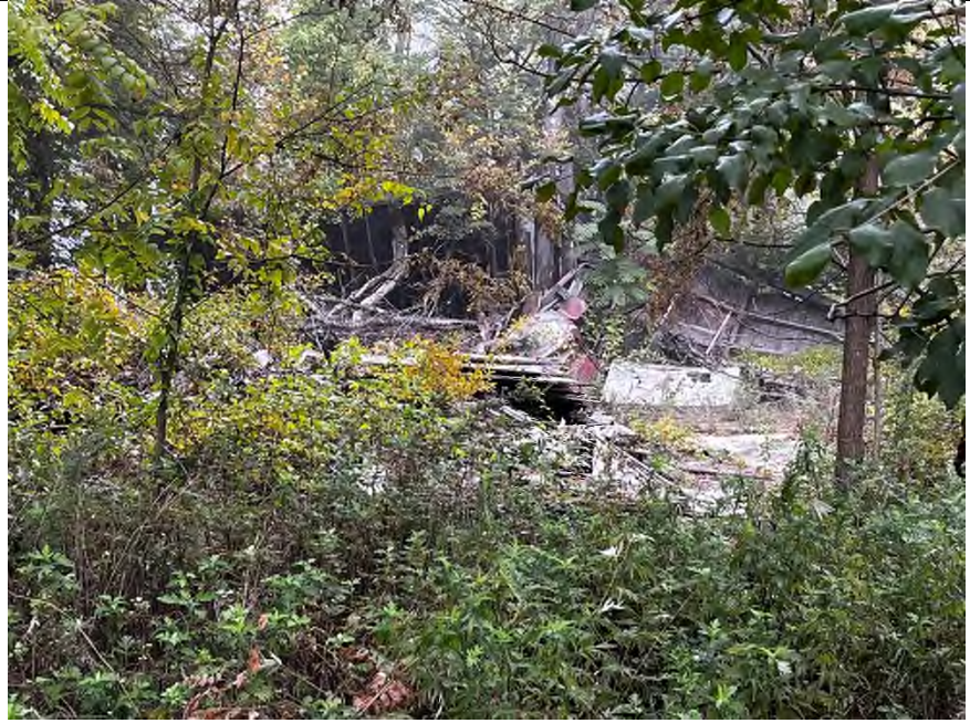
Photo 1 – Auto Garage East (Collapsed).
