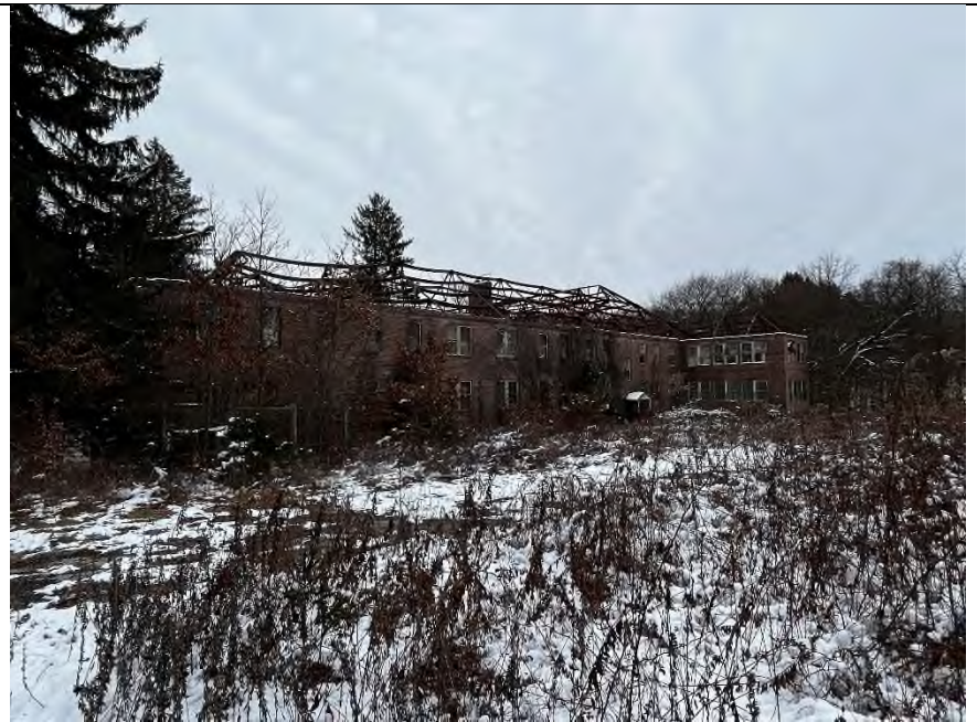
Photo 16 – Brookside structure, severe deterioration of roof.
