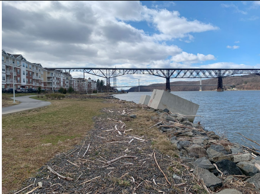
Photo 4: View of where the cap meets the Hudson River, facing south
