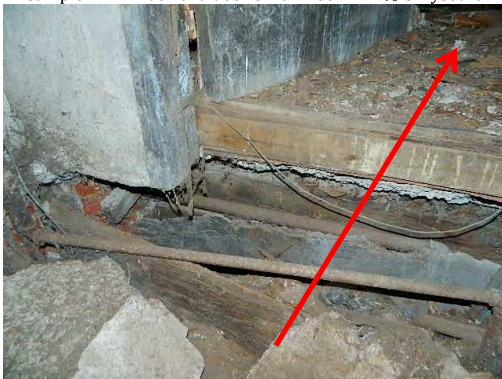
Sample# 30 – Back end debris near stairs – 80.0% Chrysotile
