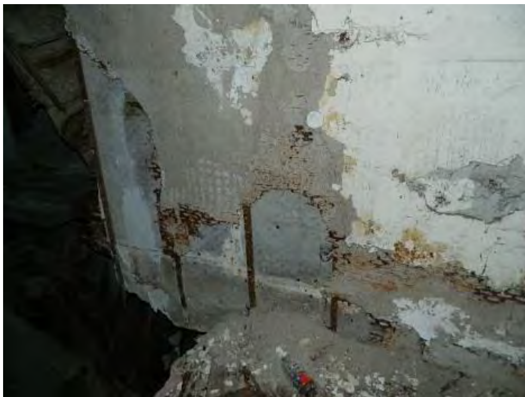
Sample# 8 – Plaster base coat – 1.5% Chrysotile
