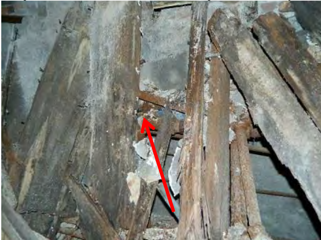
Sample# 24 – Debris at pipe right side – 1.8% Chrysotile
