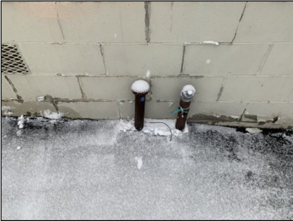
One (1) unknown capacity UST on western side, with fill port and vent line.
