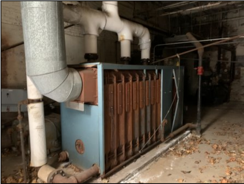
Cast iron boiler in eastern section.
