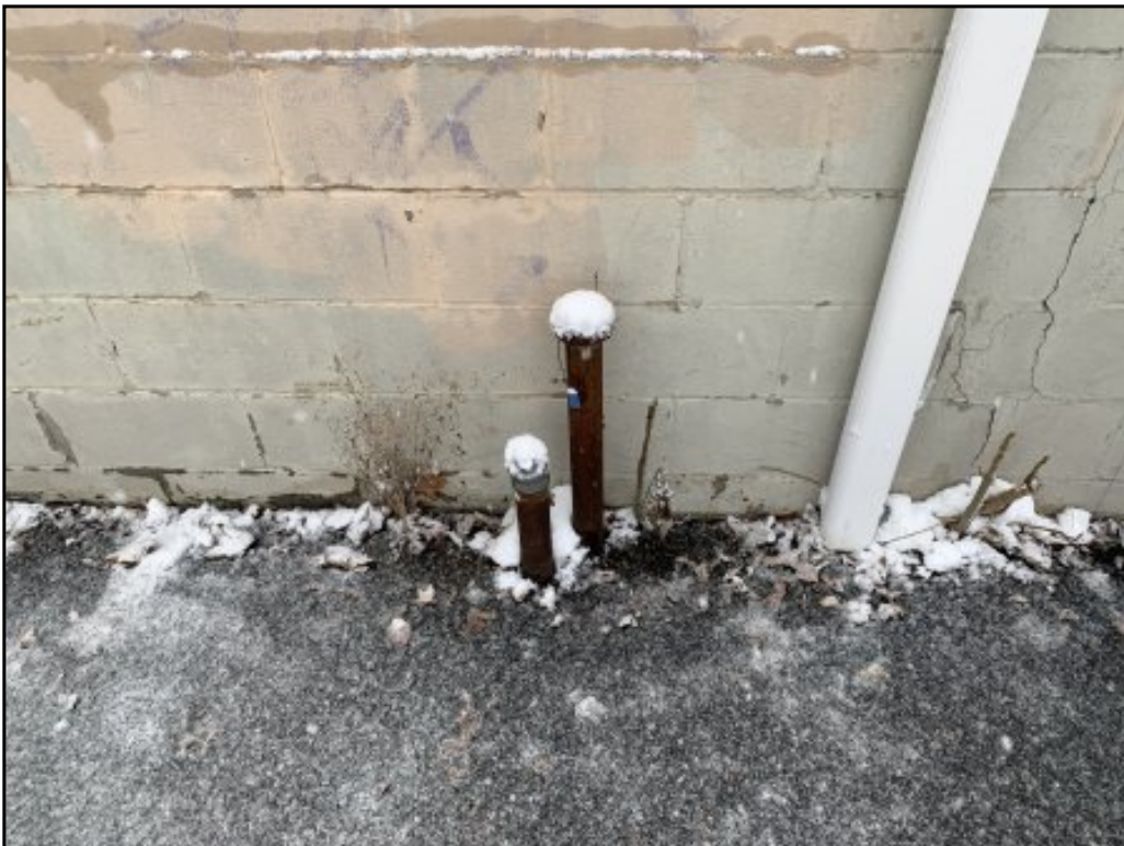
One (1) unknown capacity UST on southern side, with fill port and vent line.
