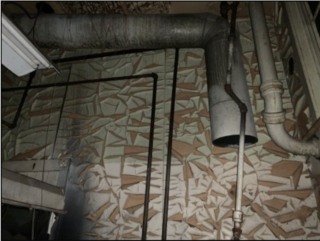
Open vent from heat treating equipment.
