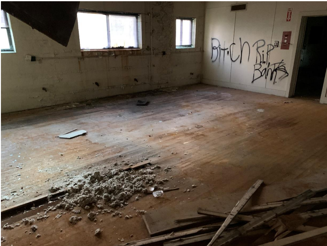
(ACM Blown-In Insulation Inside Ceiling Soffit and on Wood Floor)
