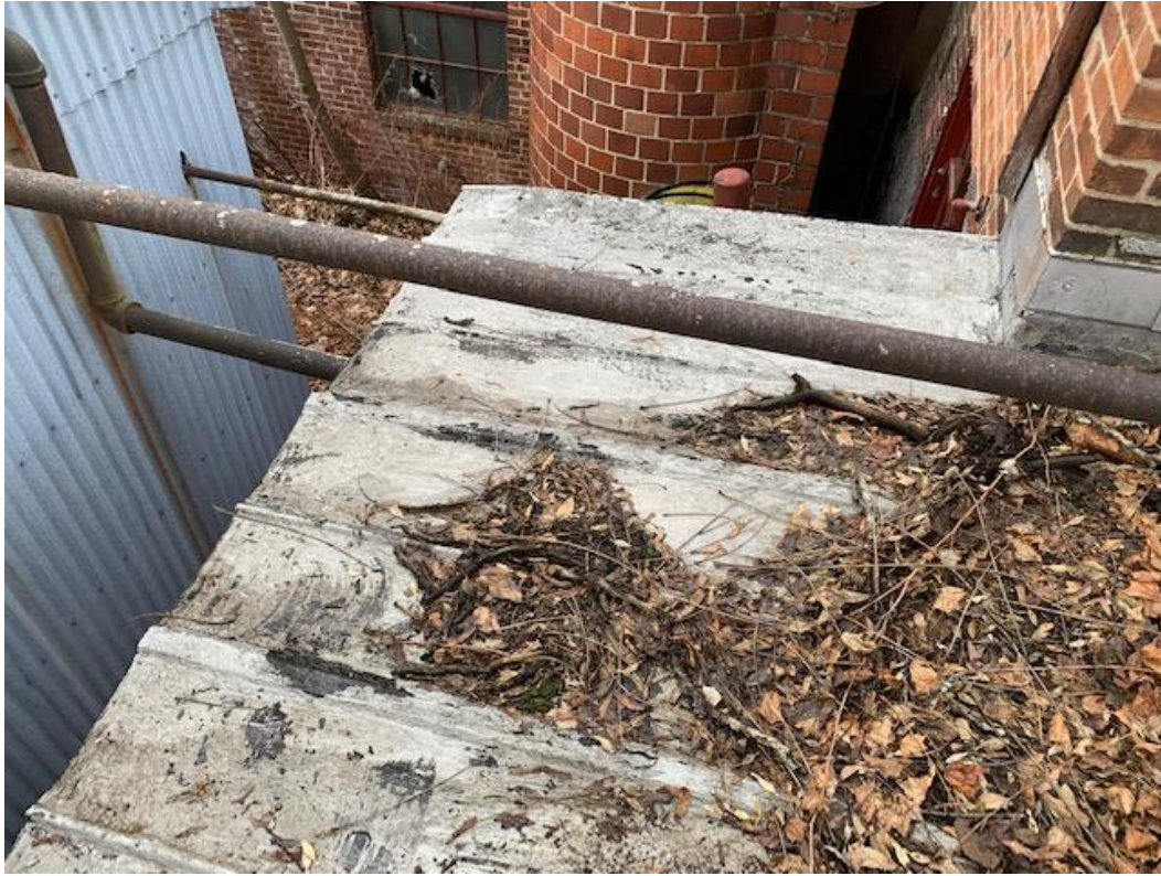
(Roof 7, ACM Tar Roofing on Metal Deck)
