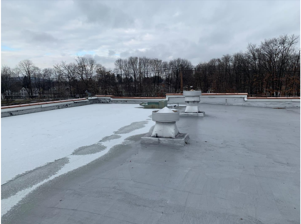
(Roof 1, ACM Flashing Tar- Parapet Wall, Equipment, Perimeter Flashing under Rolled Roofing)
