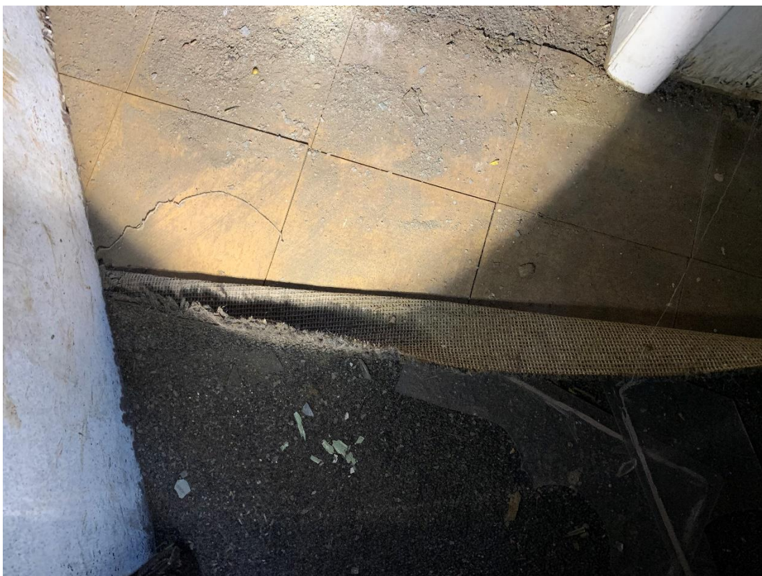
(ACM 9" x 9" Floor Tile & Mastic Under Carpet)
