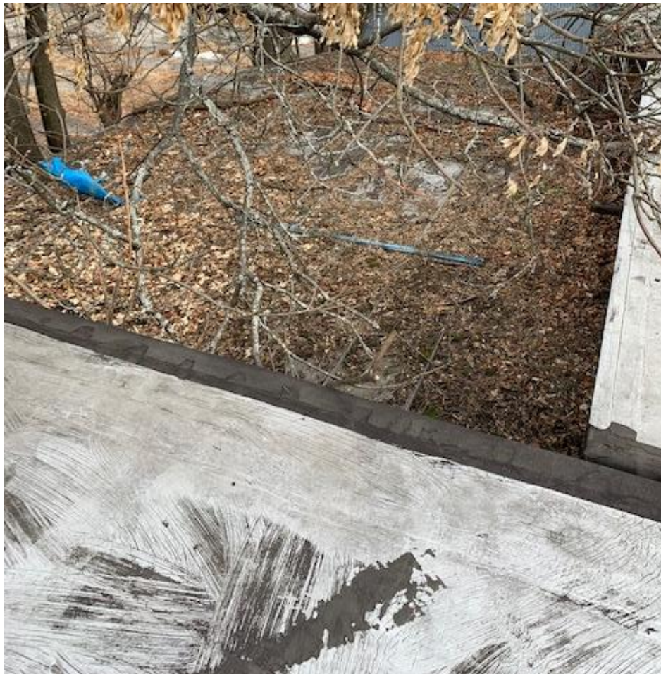
(Roof 6, (Circled) Field & Perimeter, ACM Rolled Roofing on Wood)
