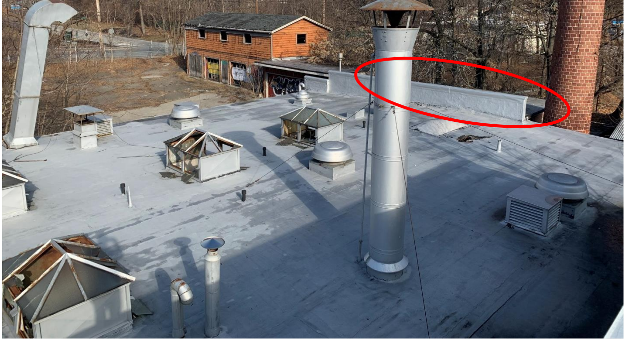
(Roof 6, (Circled) Field & Perimeter, ACM Rolled Roofing on Wood)
