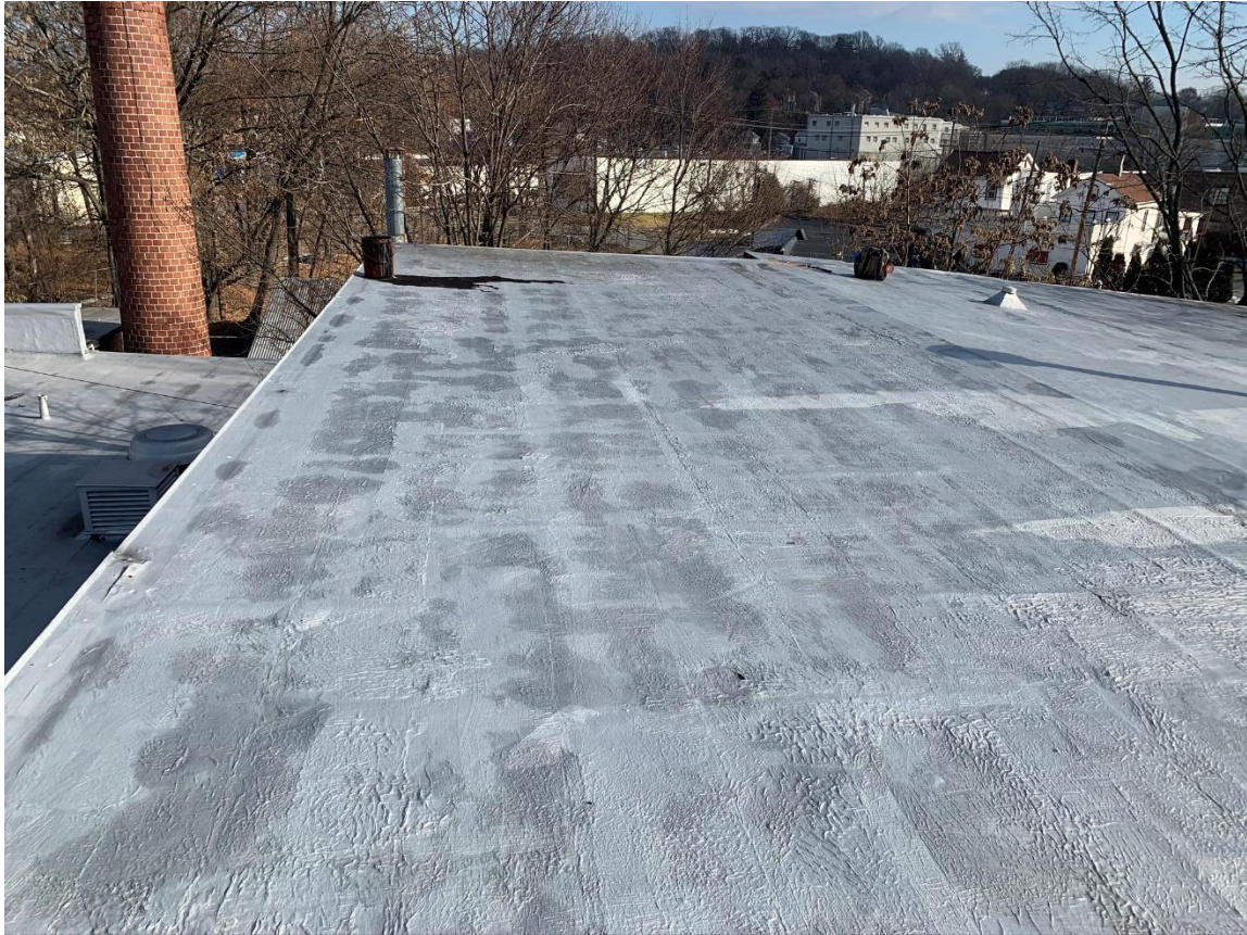
(Roof 4, Flat Side, Top Layer ACM Tar Roofing)
