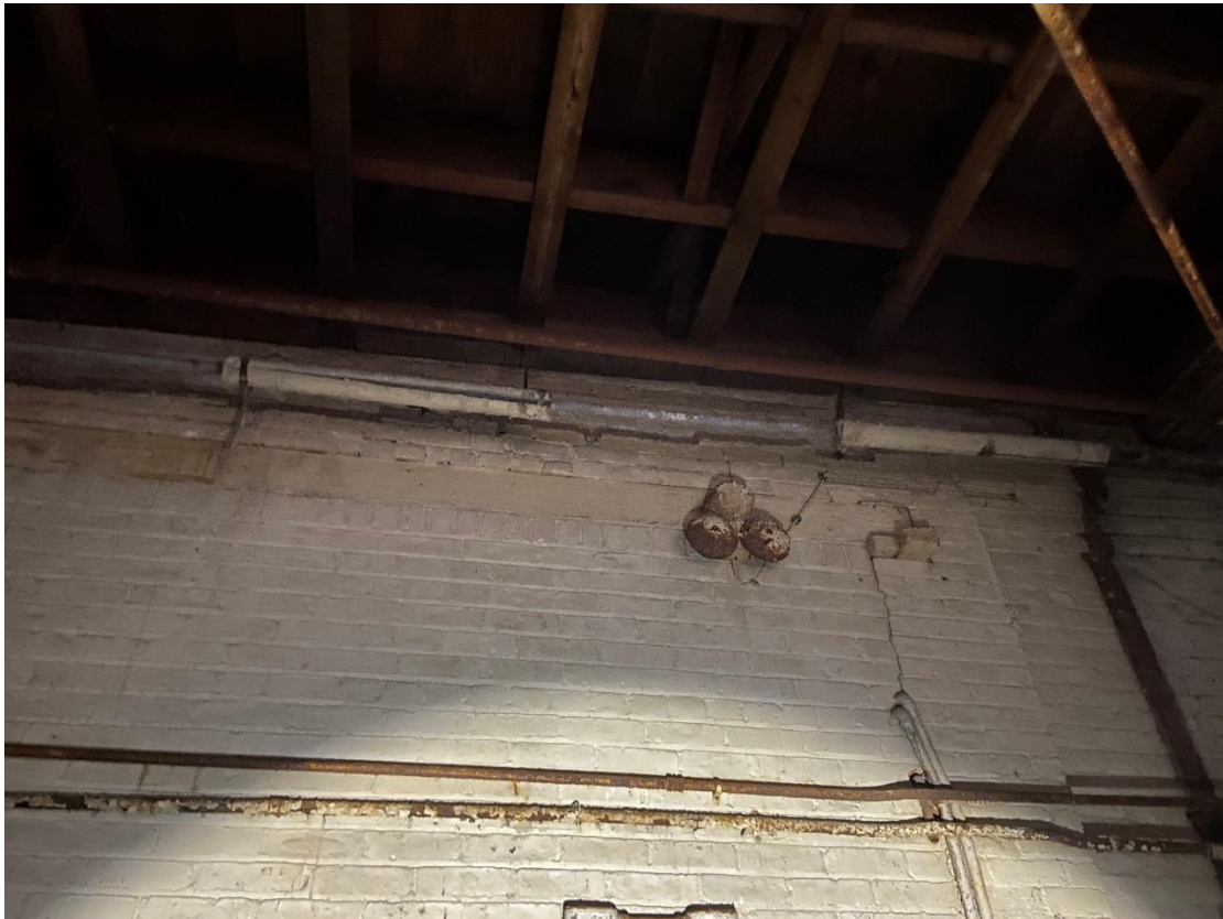
(Significantly Damaged Pipe Insulation/Mudded Joint Packing with Debris on 1 st Floor)
