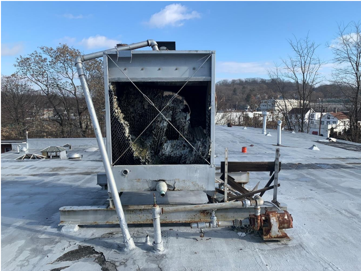
(Significantly Damaged ACM Vent Filters on Roof 1 & 3)
