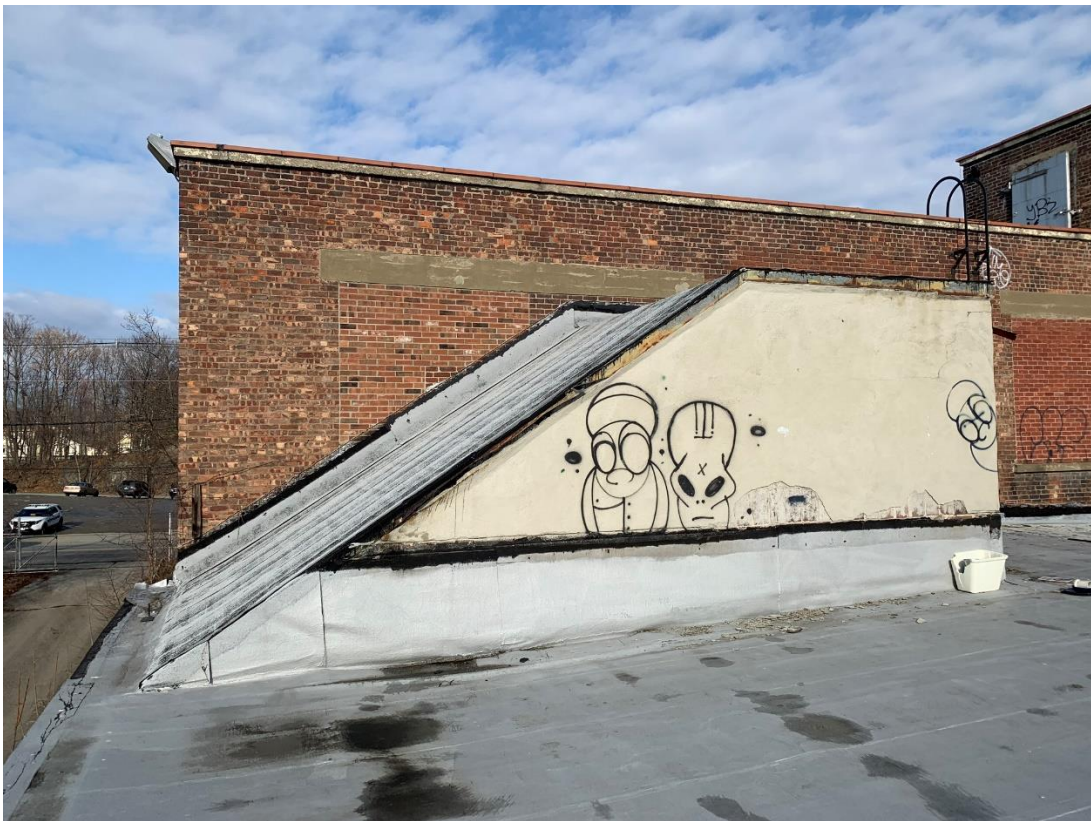
(Roof 3, Stair Tower Roof, Bottom Layer ACM Built-Up Roofing, on metal)
