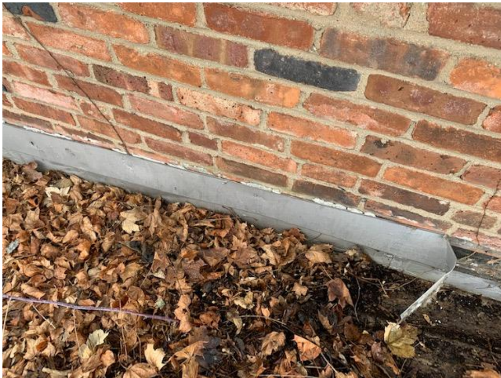
(Roof 7, Flashing to Roof 6, ACM Caulk on Brick & Metal)
