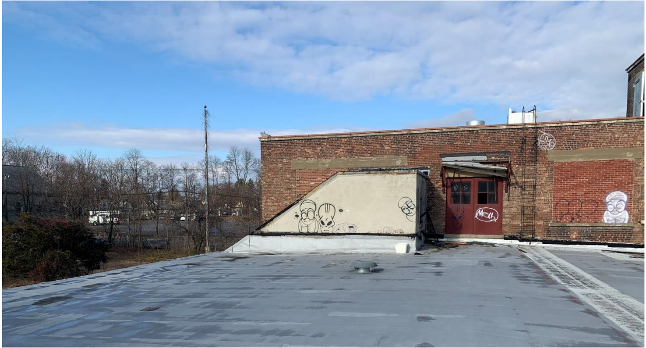
(Roof 3, Building ACM Flashing Tar, On Brick and Stucco, Bottom Layer)
