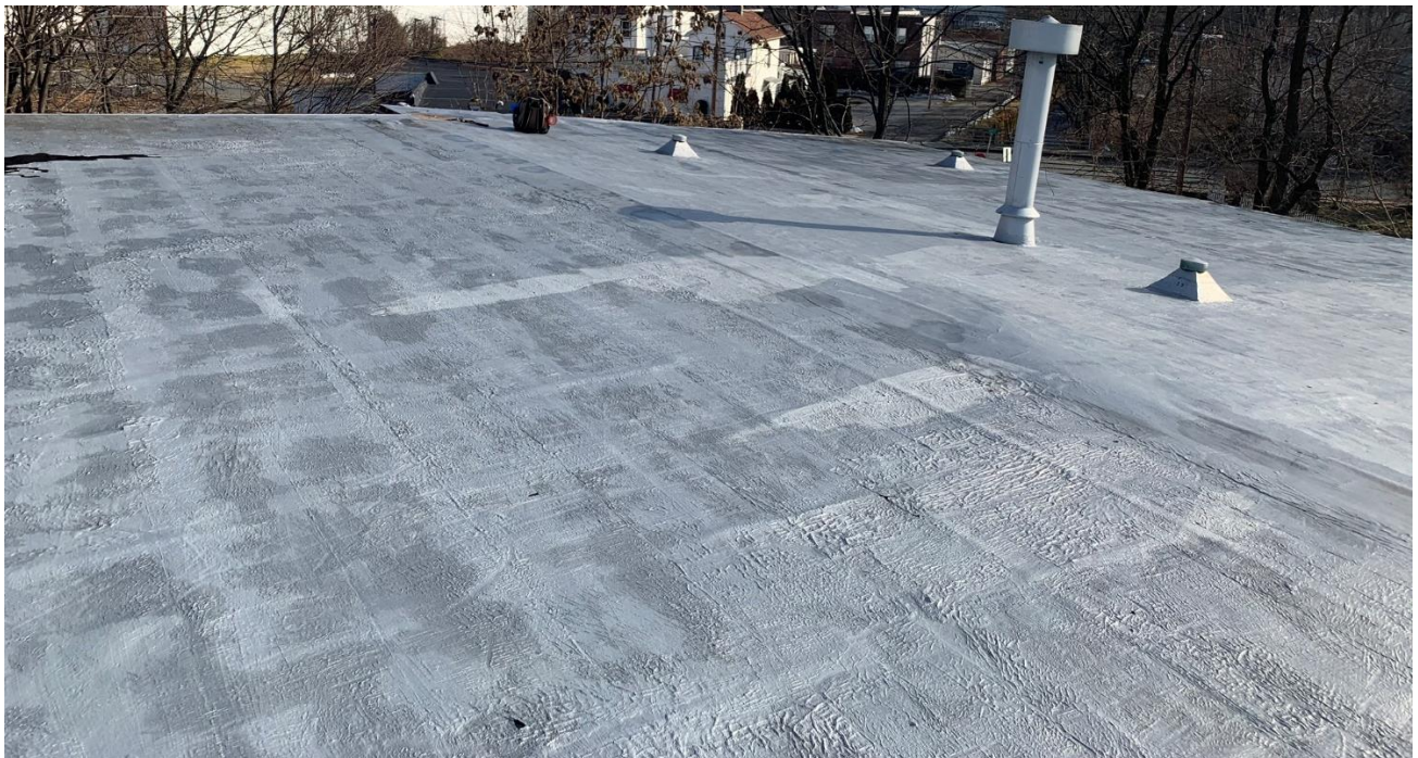
(Roof 4, Pitched Side, 3 rd Layer, ACM Vapor Barrier)
