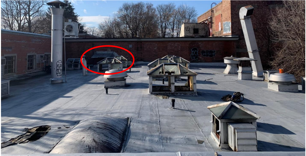
(Roof 5, Dormer Roof (Circled), Building & Equipment ACM Flashing Tar)
