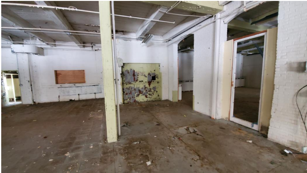
Picture 1.0: Lead-Based White Wall Paint on Bricks, Lead-Based Paint on the Elevator Door, Lead-Based Paint on the Columns in the Warehouse of Building 1.
