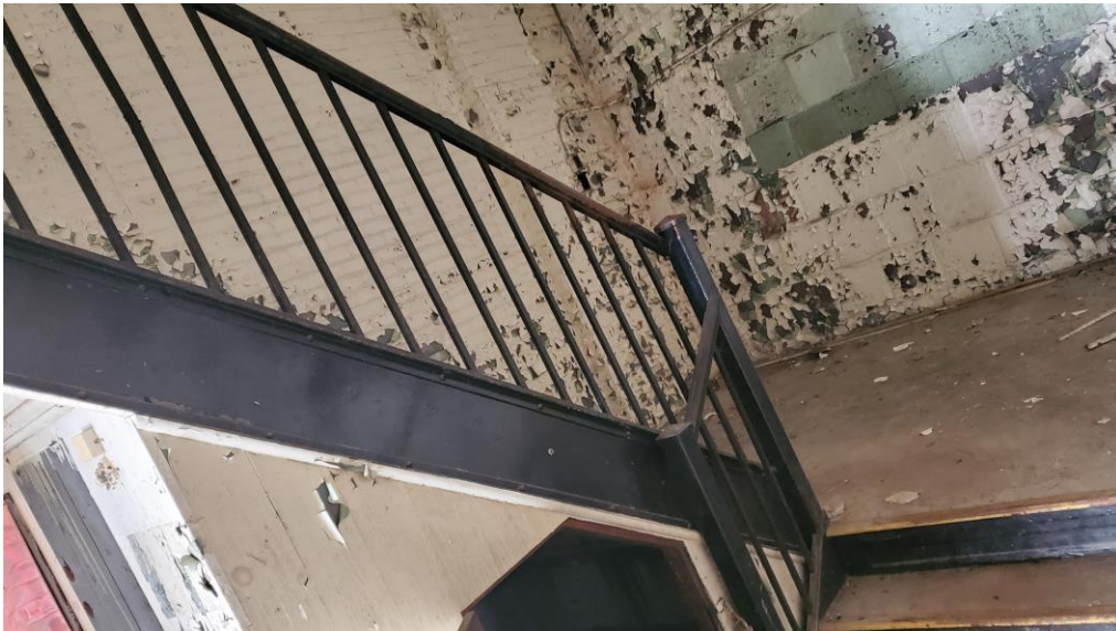
Picture 4.0: Lead-Based Paint on the Staircase system of Building 1.
