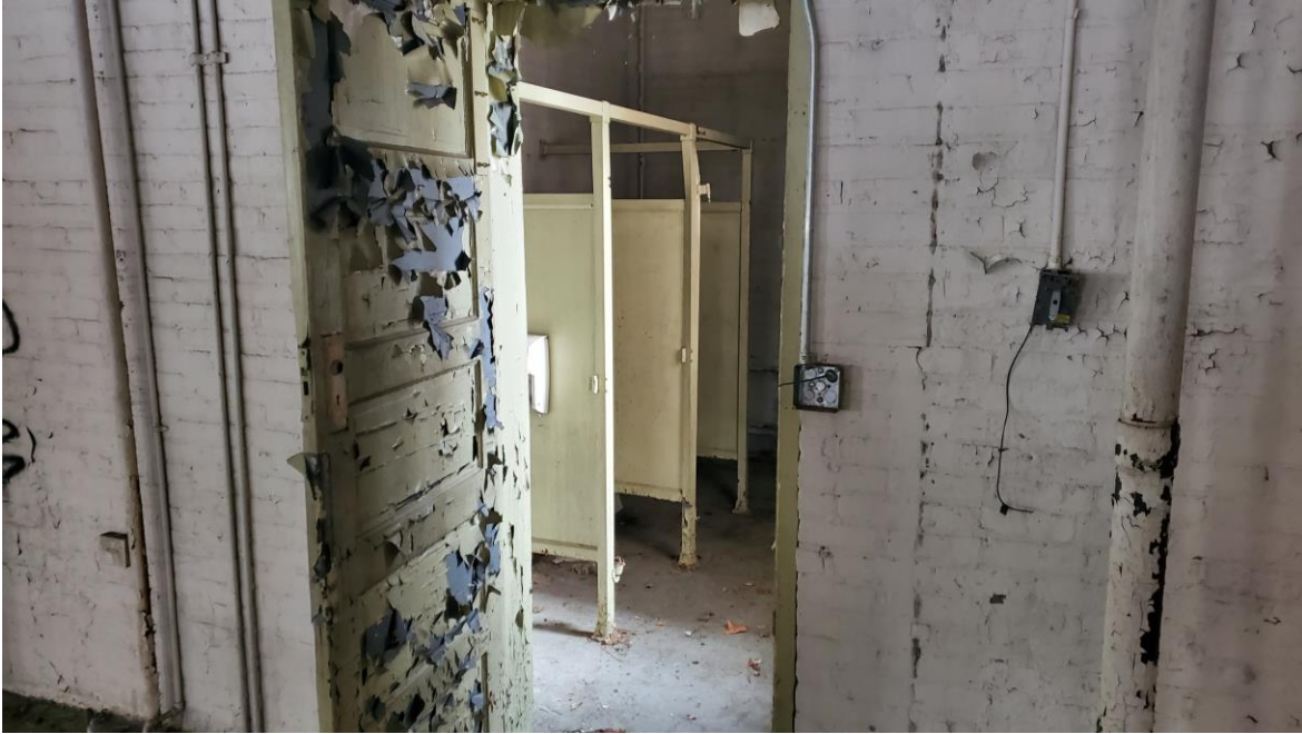
Picture 7.0: Lead-Based Green Paint on the Bathroom Doors in various parts of the different buildings.
