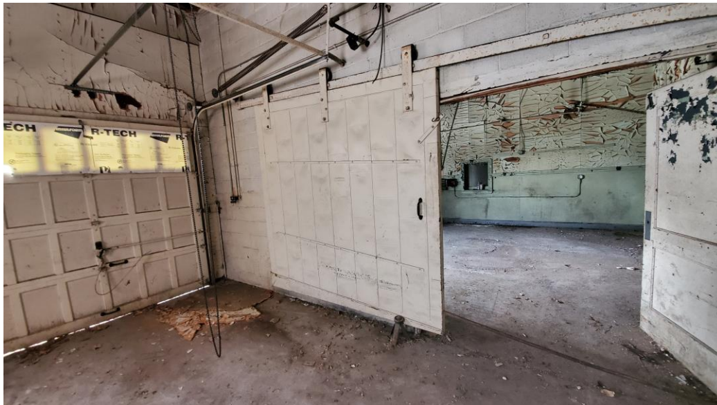
Picture 2.0: Lead-Based Paint on the Sliding Door, as well as on the wall wood covebase in Building 4.
