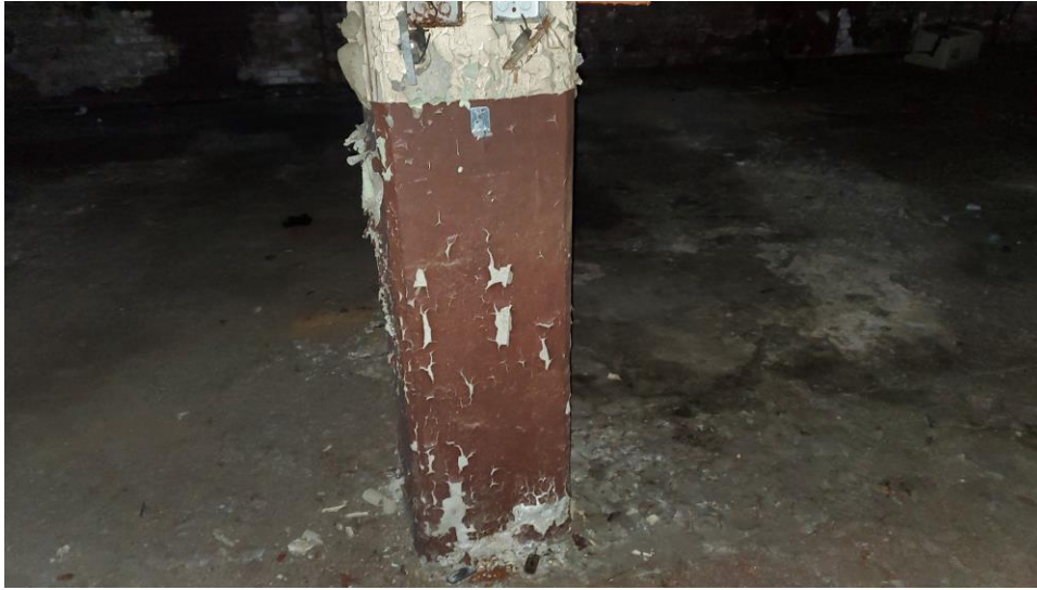
Picture 5.0: Lead-Based Brown Paint on the Columns of the Basement in Building 1.
