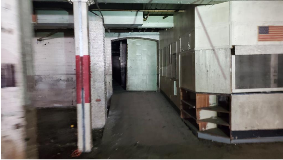
Picture 3.0: Lead-Based Paint on the Sliding Door of the Basement of Building 1 to Building 2.
