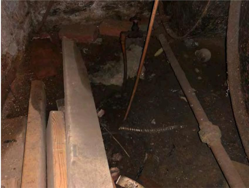
7. Partially buried fuel lines, eastern-central portion of Building A basement
