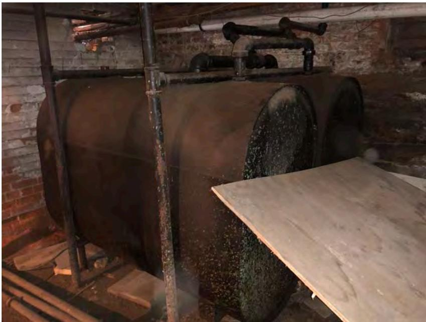
6. Two manifolded, 275-gallon fuel-oil ASTs, near eastern-central interior wall of Building A basement
