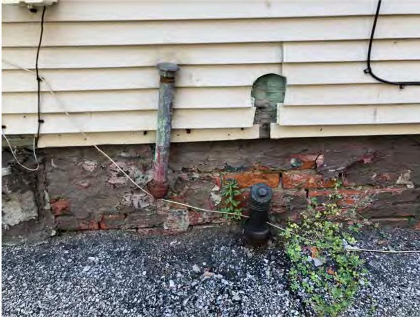
5. Fill port and vent pipe at eastern-central exterior wall of Building A, servicing an interior aboveground storage tank (AST)
