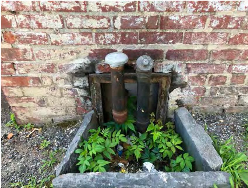
9. Fill port and vent pipe at northwestern exterior wall of Building B, servicing an interior AST
