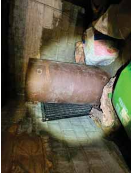
6. Discarded, empty 275-gallon tank, western portion of basement, Lot A
