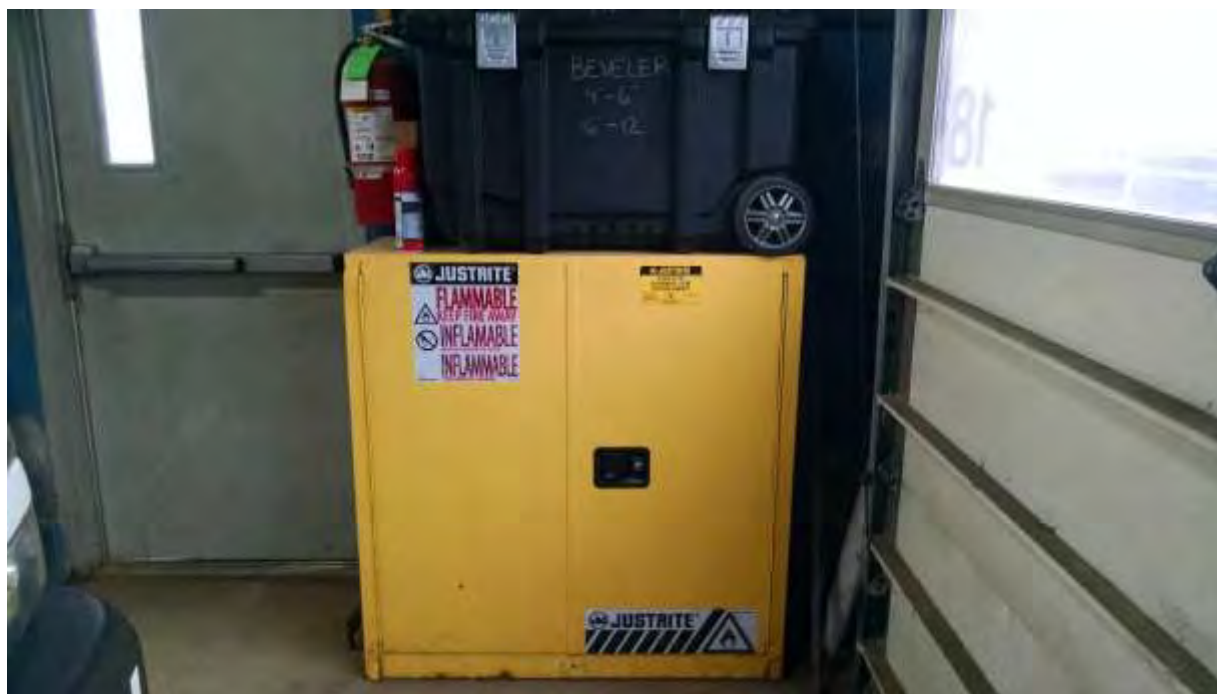
Photo 36: Flammable Liquid Cabinet - Locked
