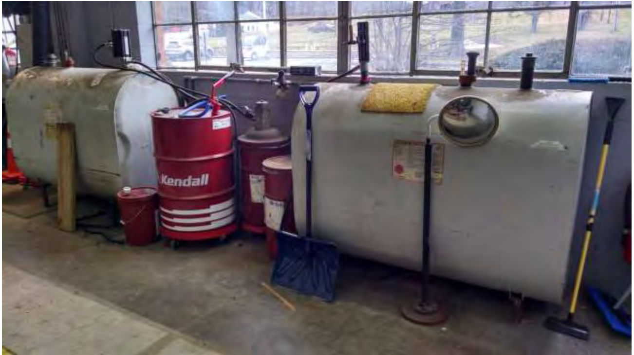
Photo 13: Waste Oil Containers (500 Gal)
