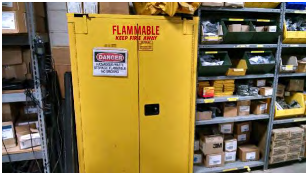
Photo 37: Flammable Liquid Cabinet – Locked
