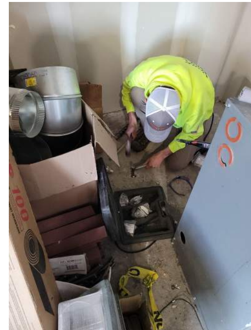
16 - Installation of T-1 Vapor Pin 04.28.2022
