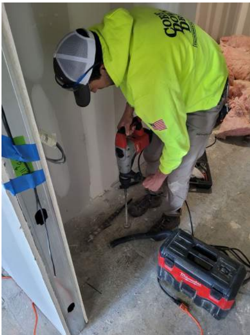
19 - Installation of T-3 04.28.2022
