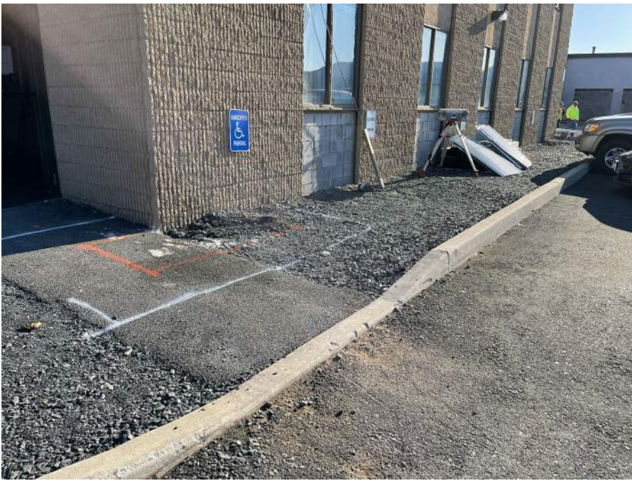
09 - Awning excavation markout 03.21.2022
