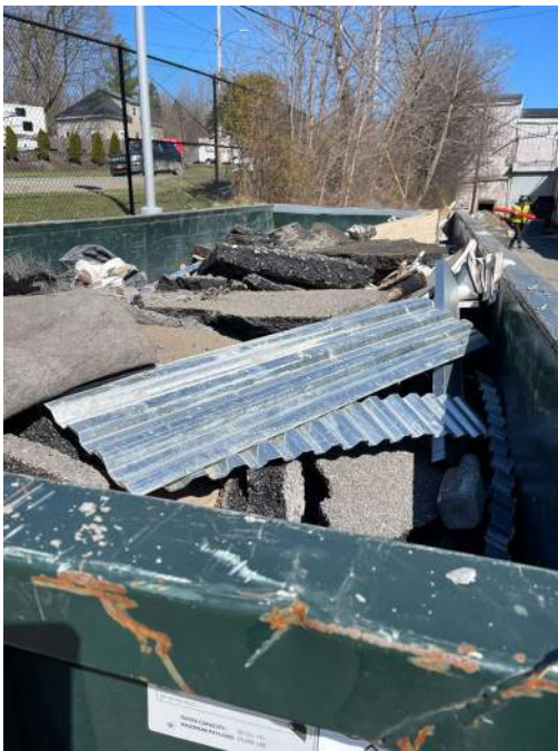
13 - Removed asphalt in dumpster 03.21.2022
