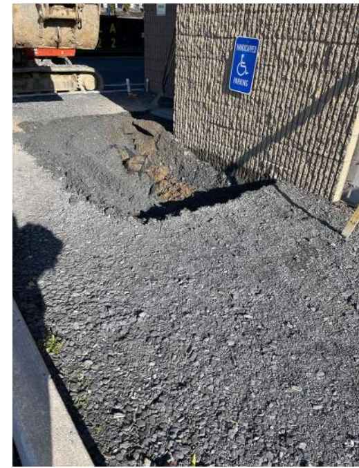
10 - Area of awning excavation 03.21.2022
