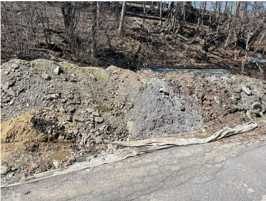
15 - Excavated soils on plastic 03.21.2022
