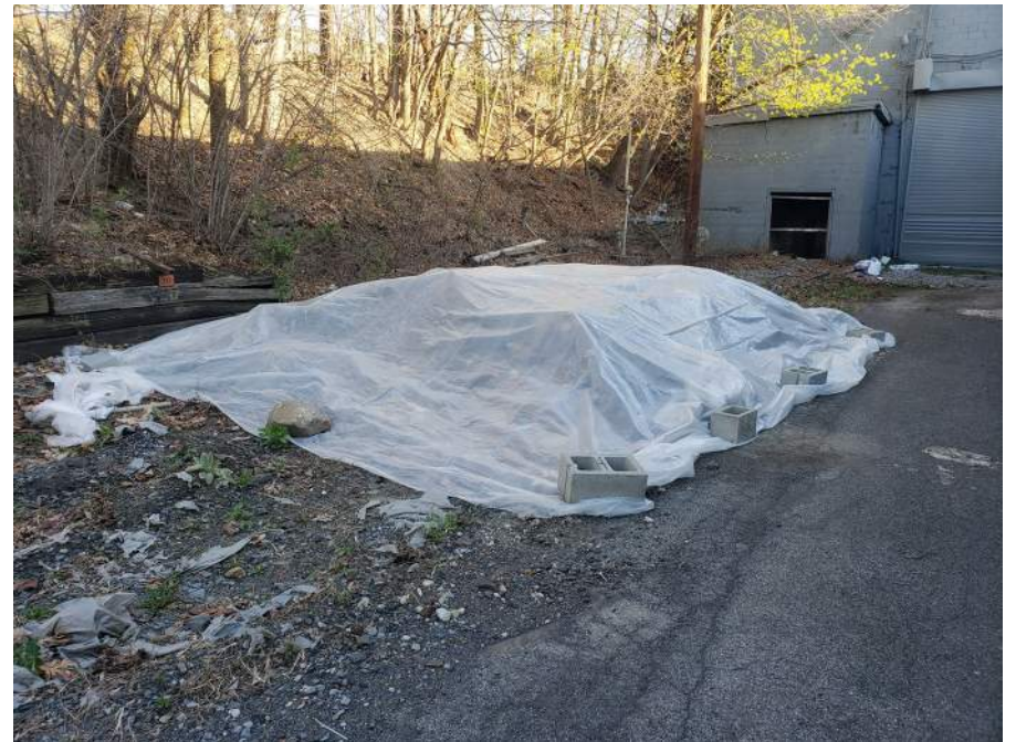
24 - Excavated Soils on Plastic 04.13.2023
