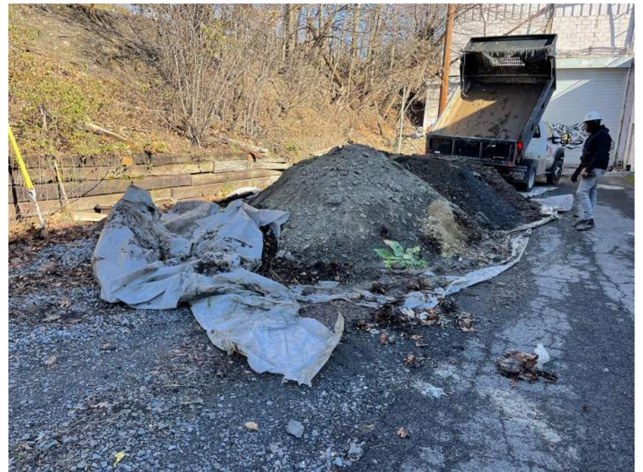
14 - Relocation of excavated soils on plastic 03.21.2022
