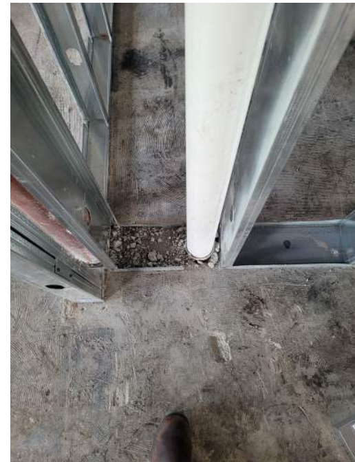
08 - SecondFloor SSDS Through Floor 02.10.2022
