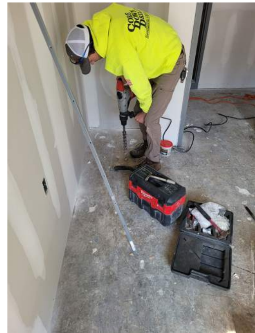
22 - Installation of T-5 04.28.2022
